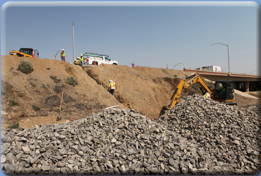
I580 Southbound Reconstruction Project
