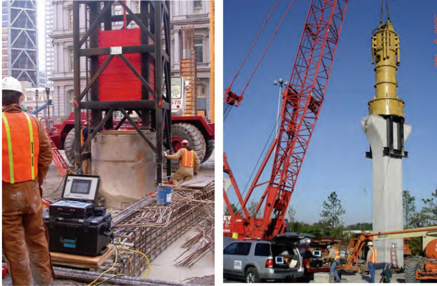
**Figure 1.13:** Example dynamic load tests on drilled shafts using a drop weight (left) and pile hammer (right) (Brown et al., 2010)
