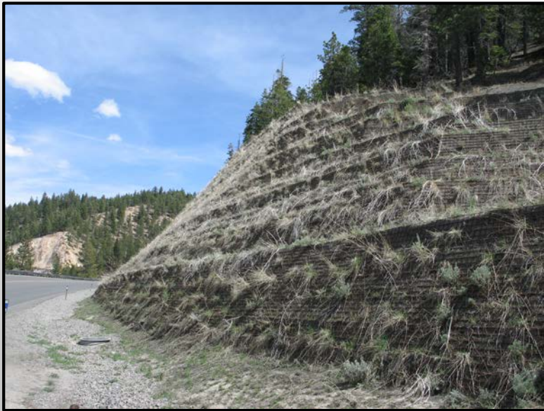
ENGINEERED SOIL SLOPE
