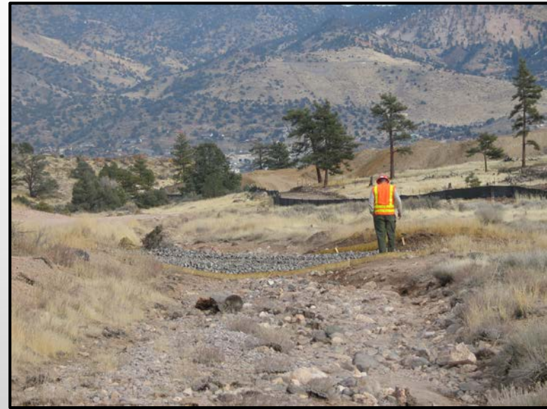
TEMPORARY STREAM CROSSING
