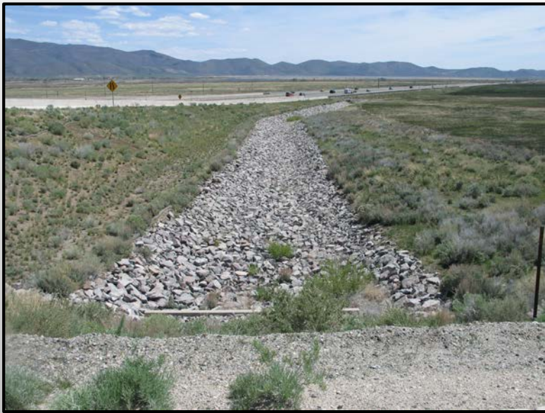
RIPRAP LINED CHANNELS
