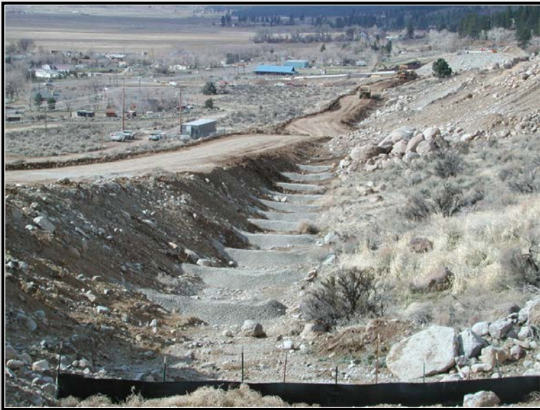
ROCK CHECK DAM
