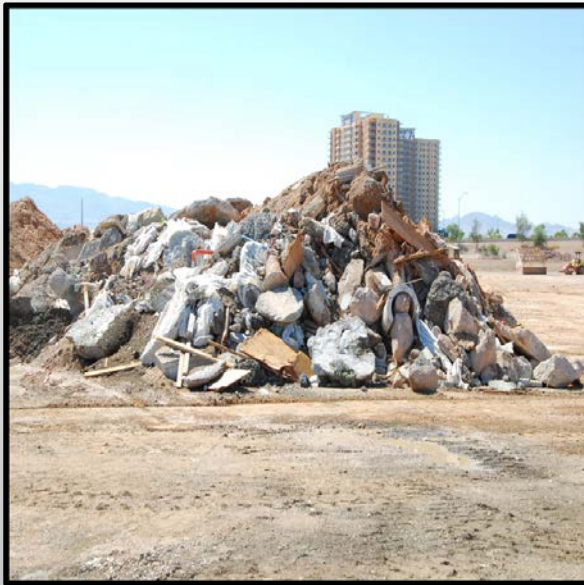
TRASH AND DEBRIS
