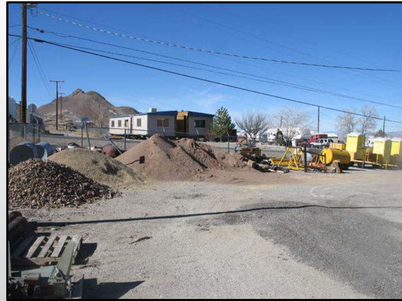
VARIOUS STOCKPILE MATERIALS
