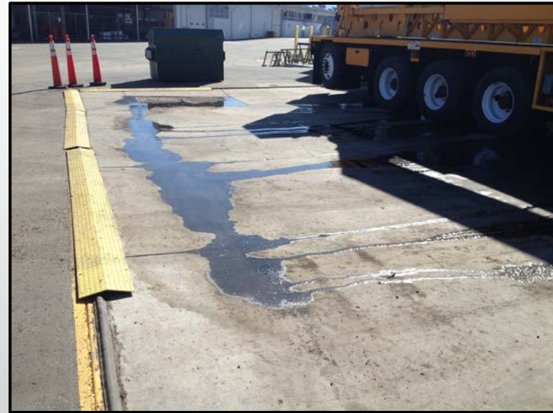
STEAM PAD DISCHARGE CONTAINMENT
