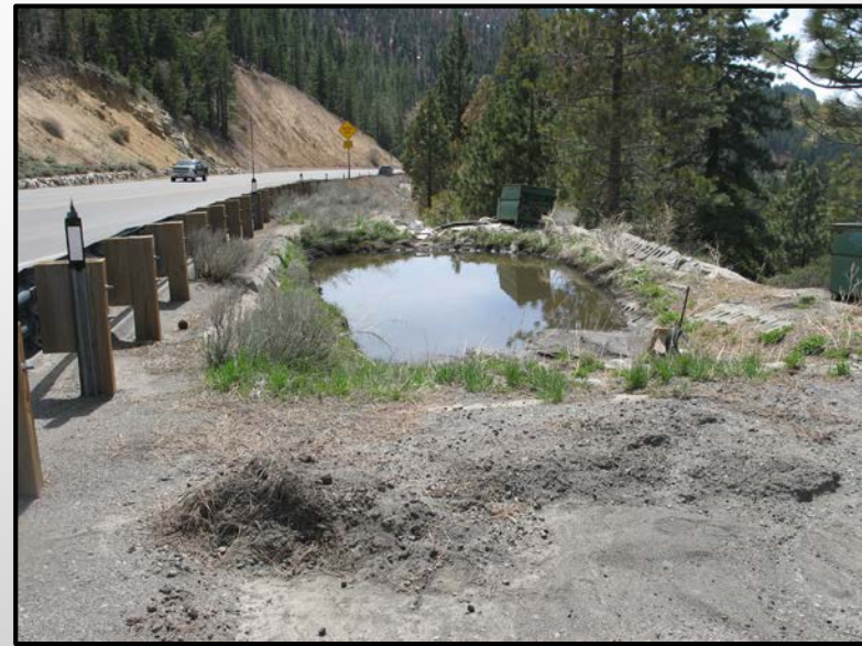
STORMWATER QUALITY BASINS
