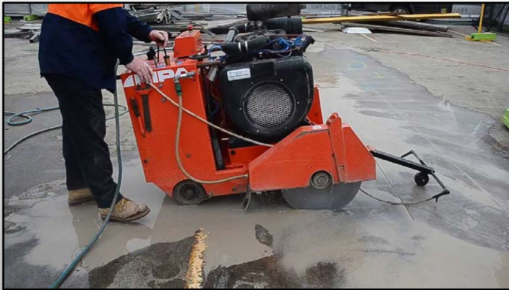
SAW CUTTING DISCHARGE
