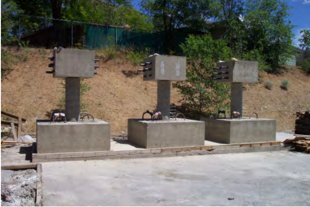
Figure 3-6 Specimen Form Removed
