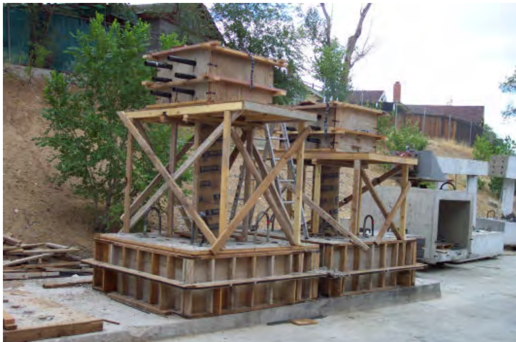
Figure 3-5 Specimen Head and Hinge Form
