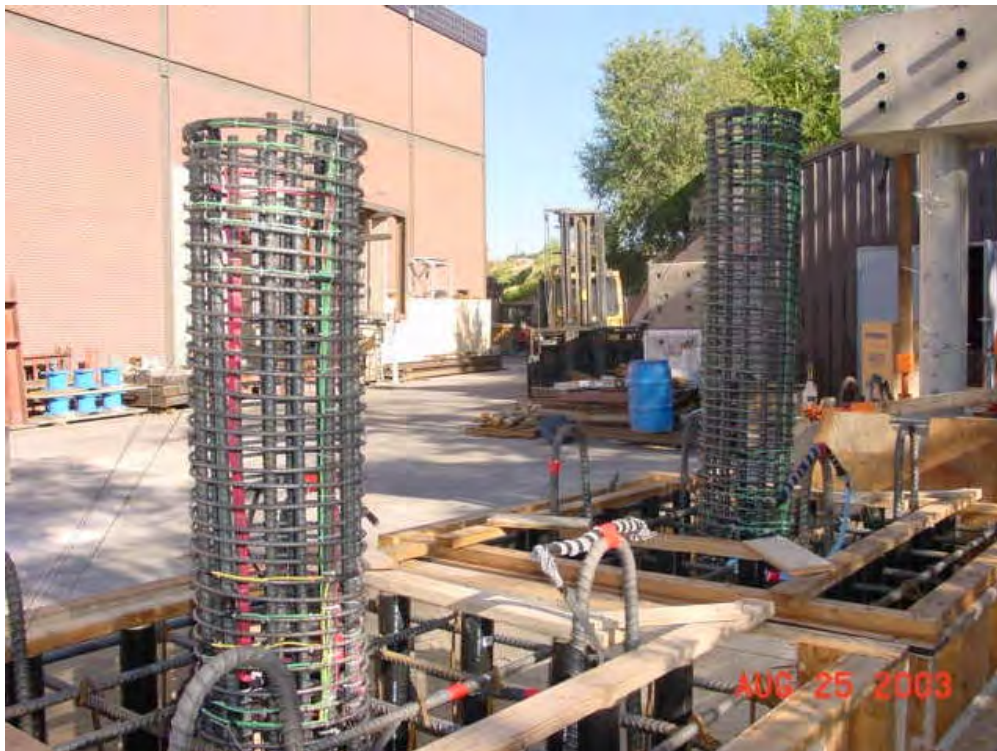
Figure 3-2 Footing Ready for Casting
