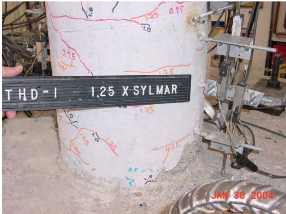
(a) Column Base
