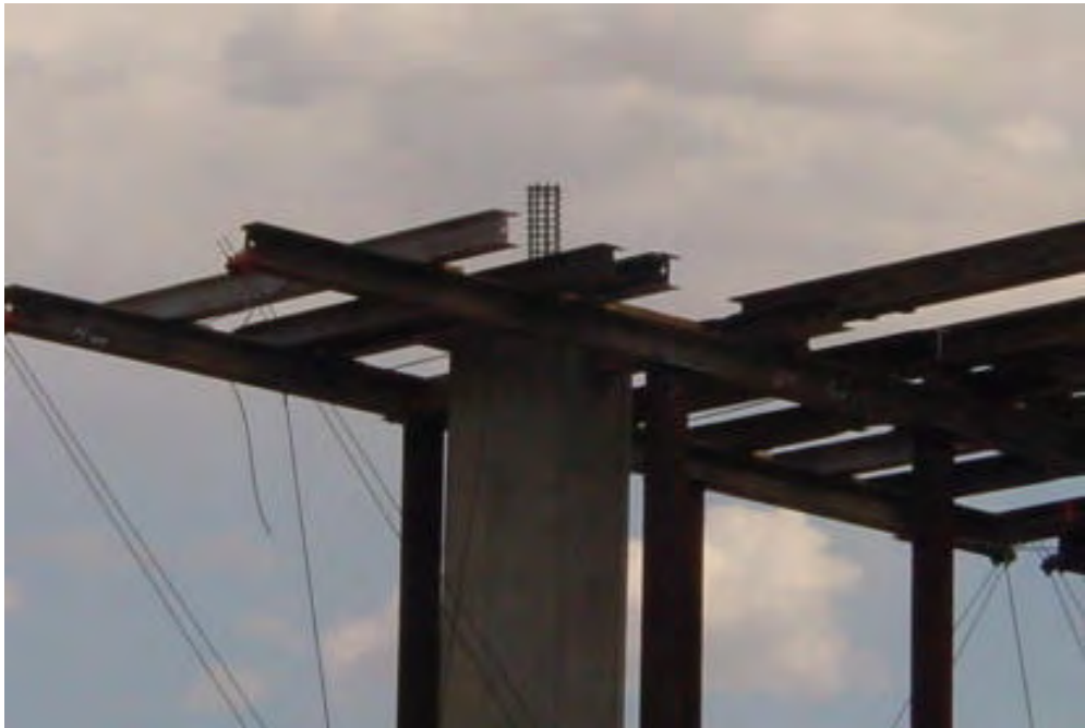
Figure 1-3 NDOT Bridge Column with Top Hinge
