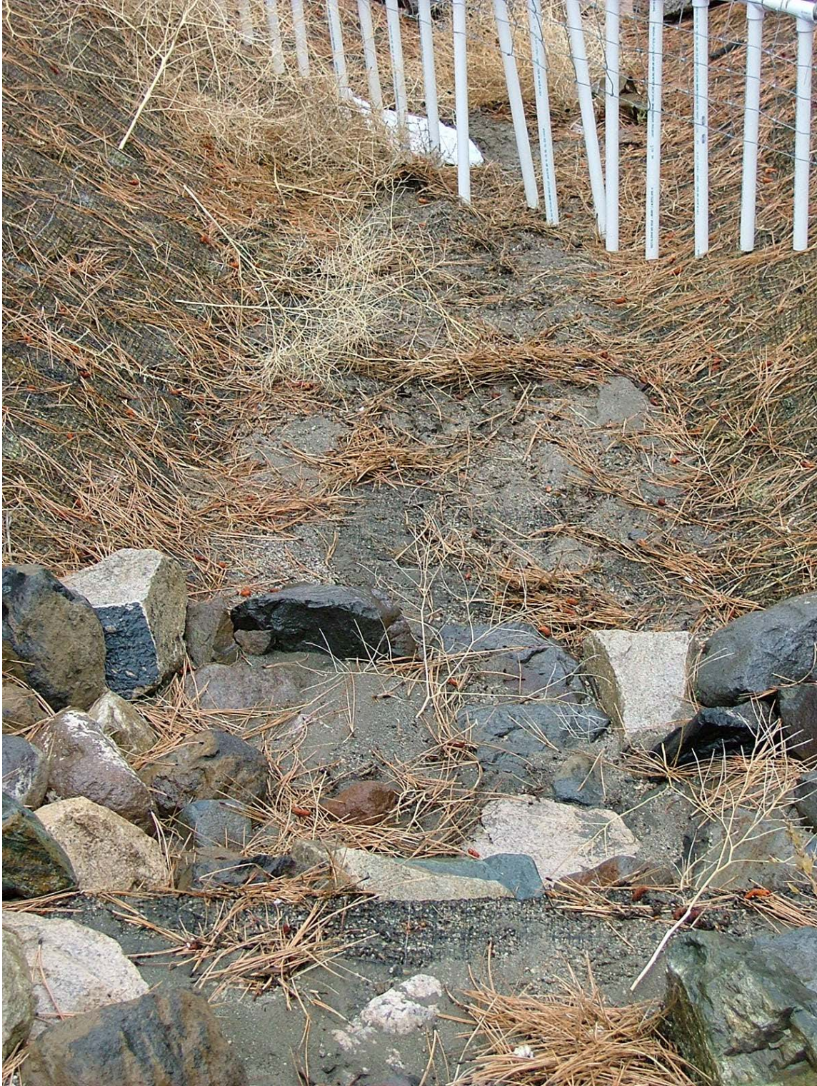
Figure 4.27 Field plot with North American Green SC250 looking downstream (November 2004).
