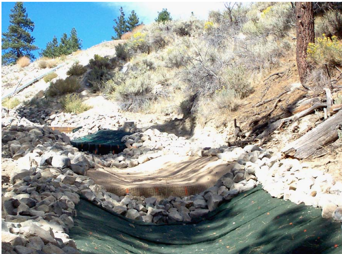
Figure 4.18 Completed installation of RECPs in upper field plots (October 2003).
