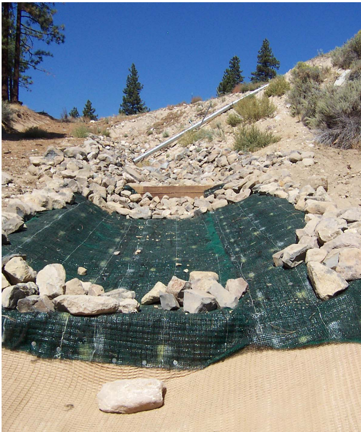
Figure 4.17 Typical channel test section after installation of RECP (September 2003).
