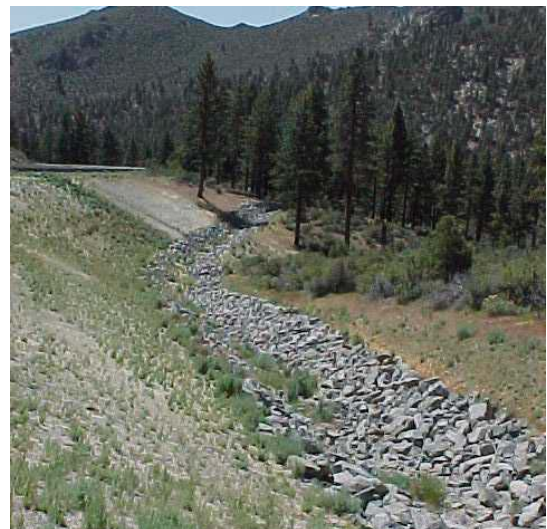
Figure 2.26 Riprap channel protection.
