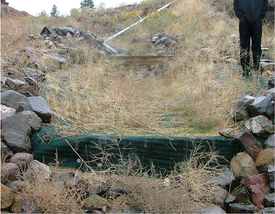
Figure 4.24 Field plot with North American Green P550 looking upstream (November 2004).
