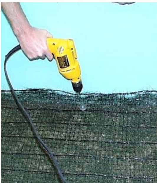
a) Anchoring TRM to Sideboard
