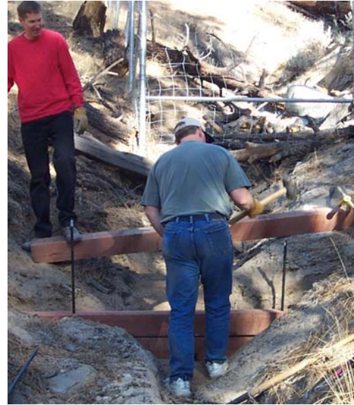
b) Steel rod anchoring of the timbers.
