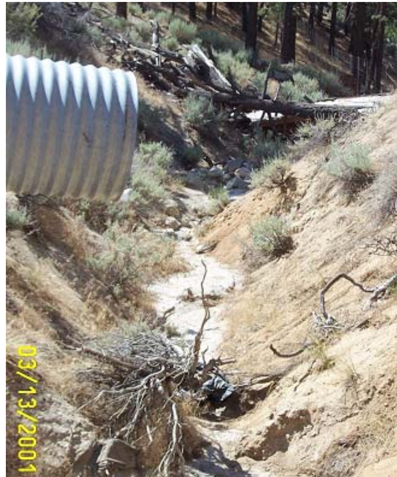
b) Looking Downstream from the Culvert Outlet
