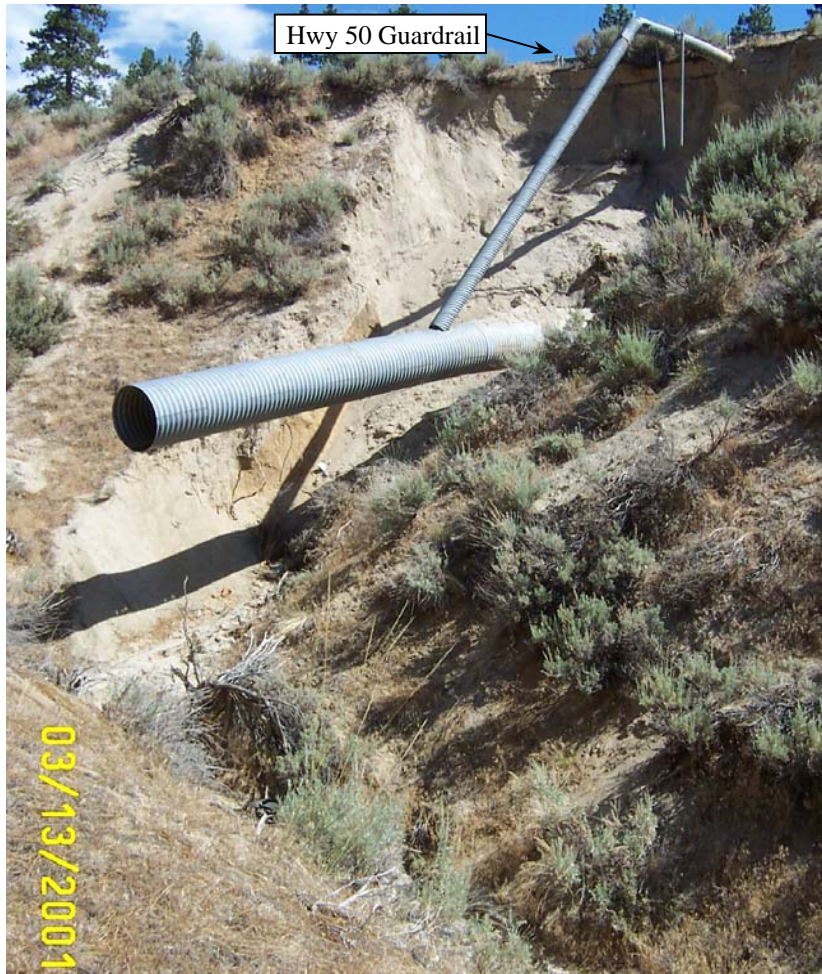
a) Looking Upstream at the 24" CMP Culvert Outlet
