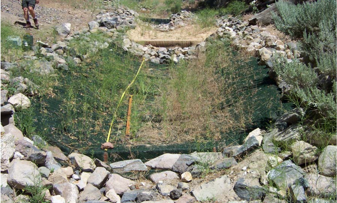
Figure 4.22 Field plot with SI Geosolutions Landlok 450 looking upstream (July 2004).
