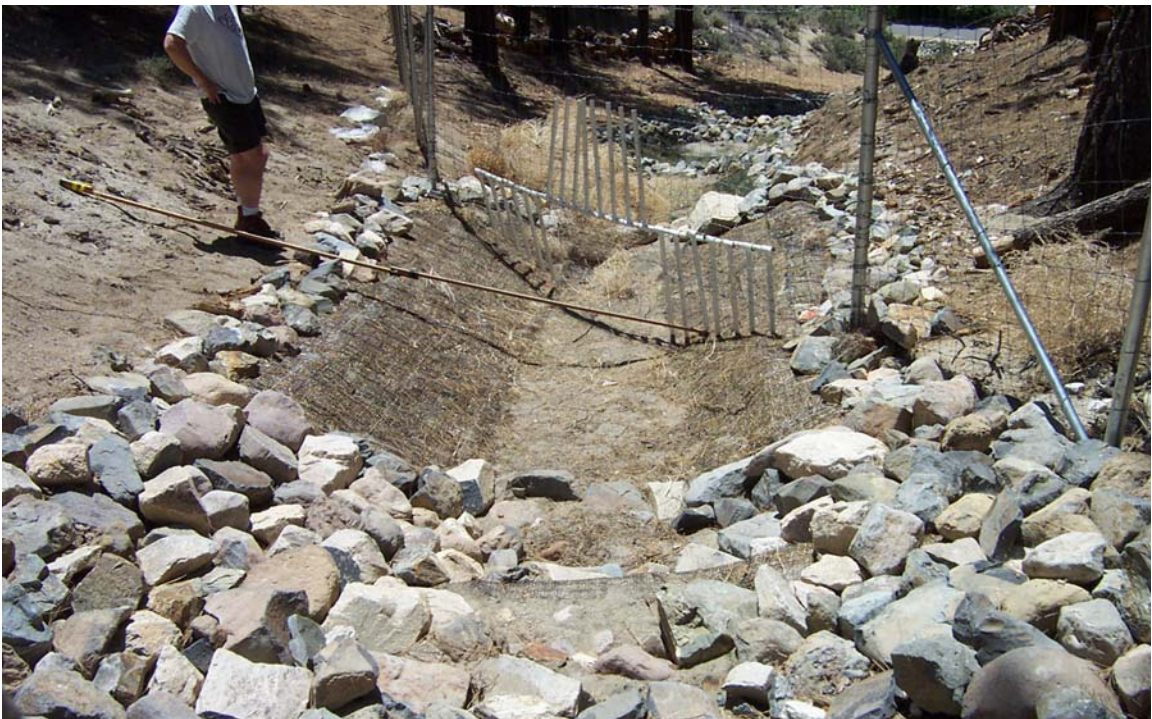
Figure 4.23 Field plot with North American Green SC250 looking downstream (July 2004).
