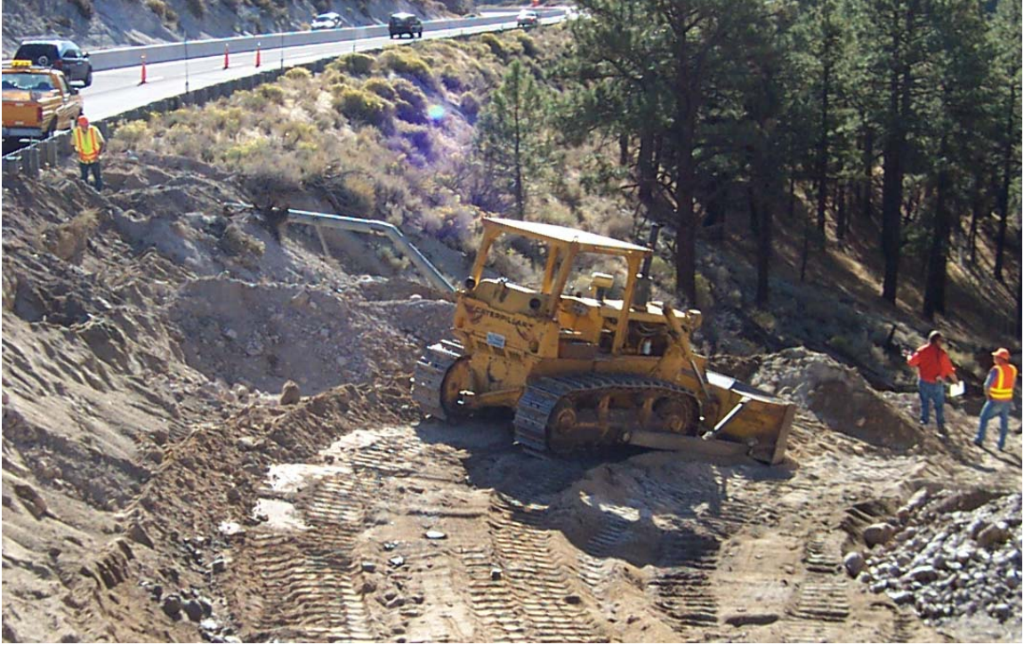
Figure 4.12 Earthwork during initial site preparation at culvert outlet (August 2002).
