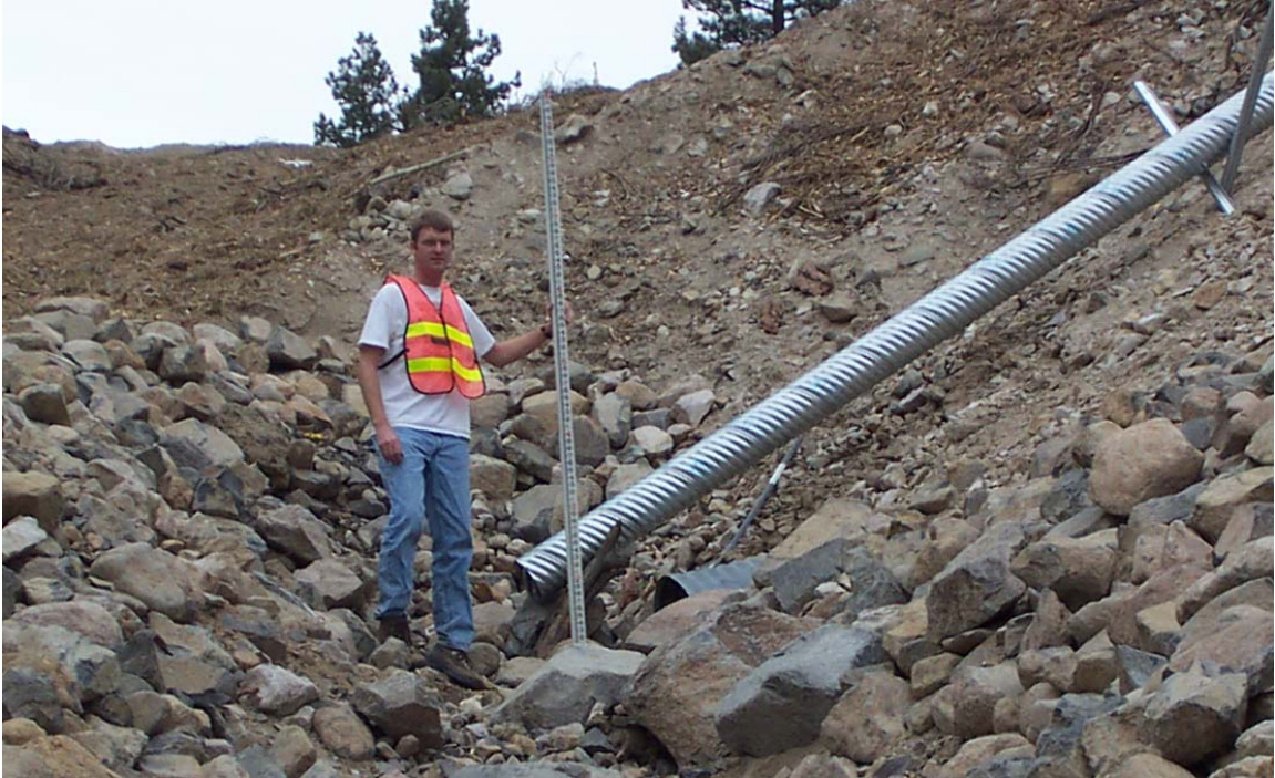
Figure 4.13 Reconstructed culvert outlet (September 2002).
