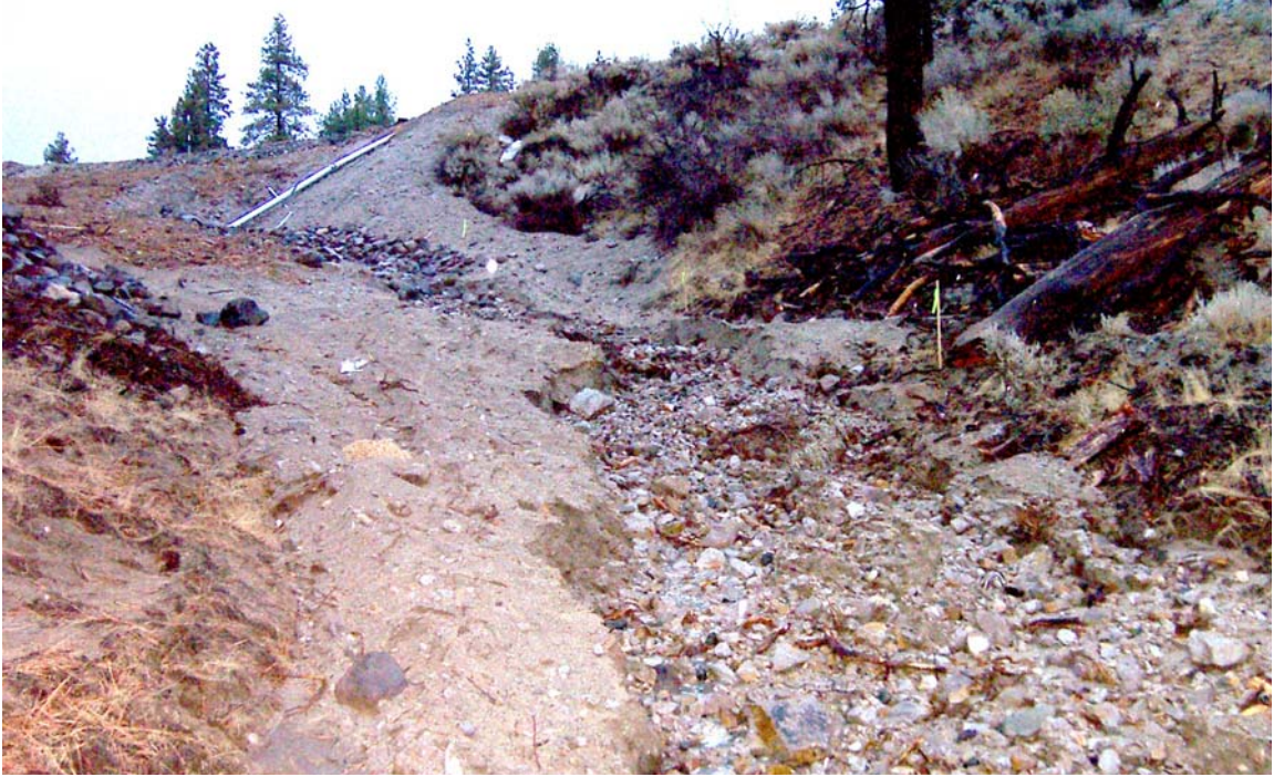
Figure 4.14 Initial site preparation after storm (October 2002).
