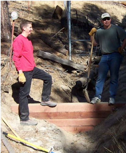
c) Completed timber drop structure.
