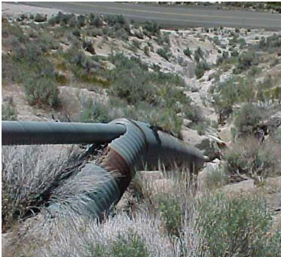
Figure 2.23 Culvert with free discharge.
