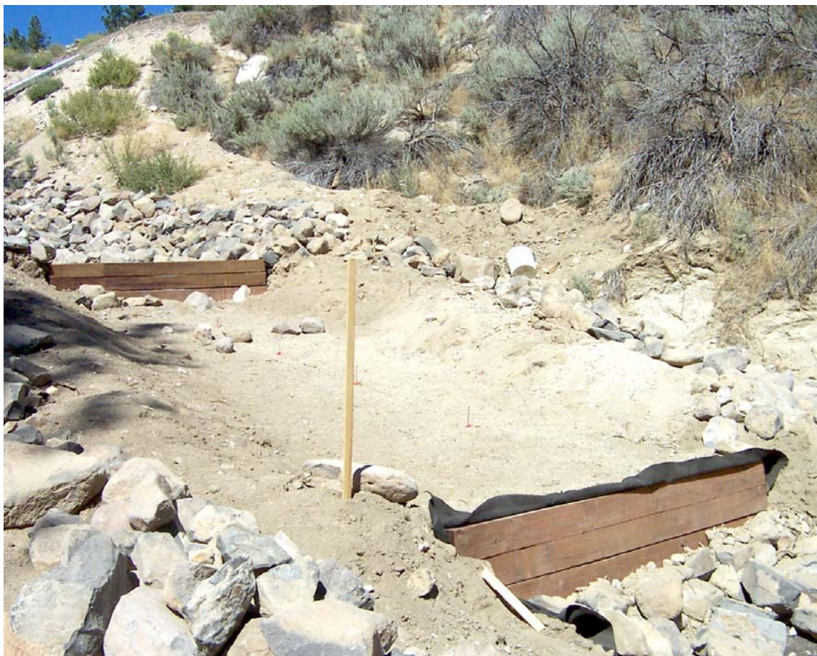
Figure 4.16 Typical channel section of field plot before installation of RECP (August 2003).
