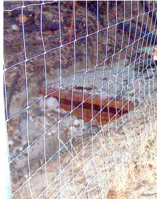
d) Backfilled by erosion upstream.
