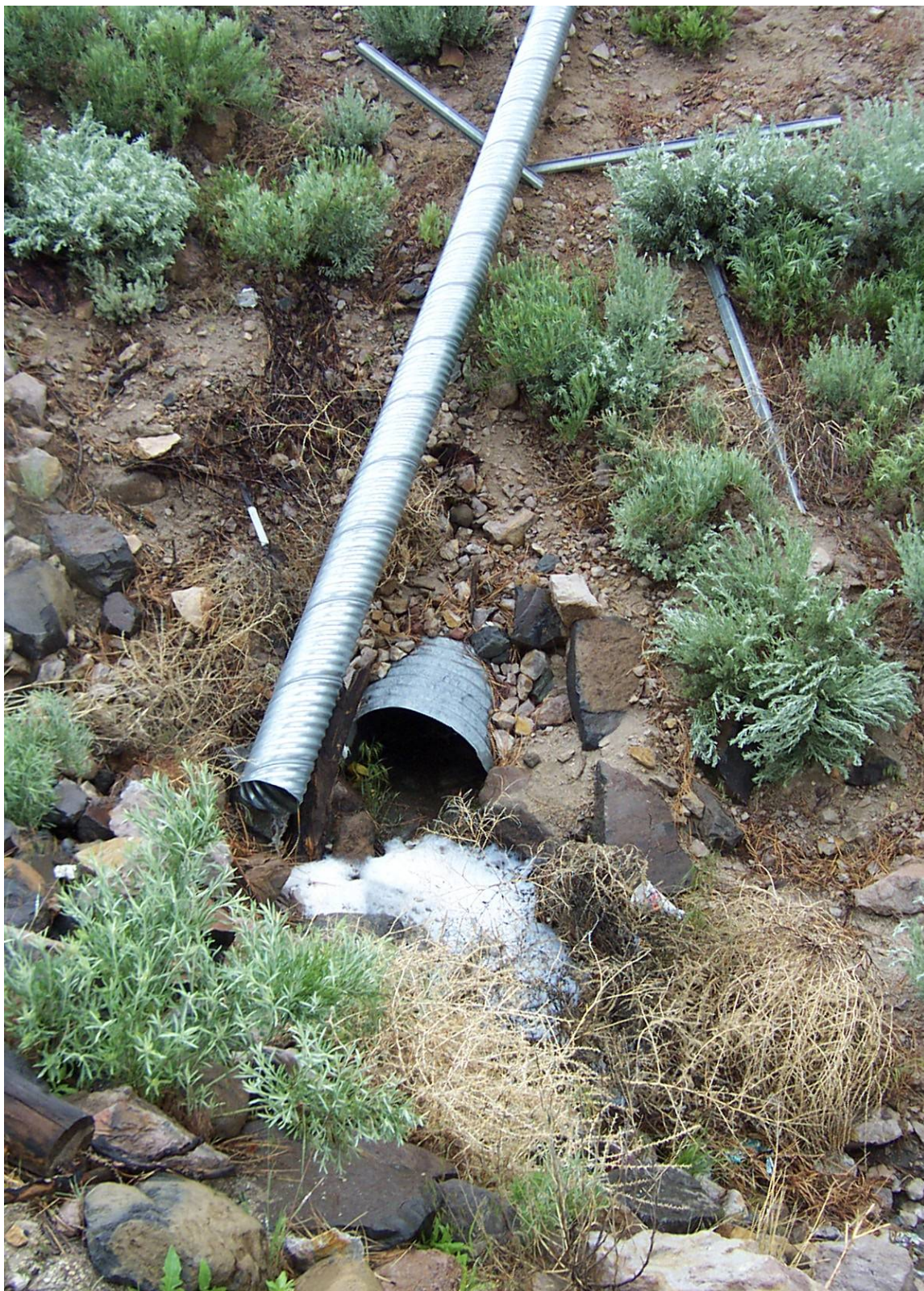
Figure 4.28 Culvert outlet (June 2005).
