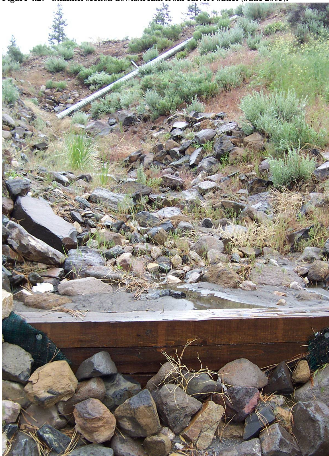
Figure 4.29 Channel section downstream from culvert outlet (June 2005).
