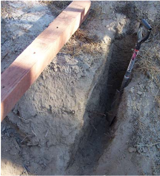
a) Key trench for timbers.
