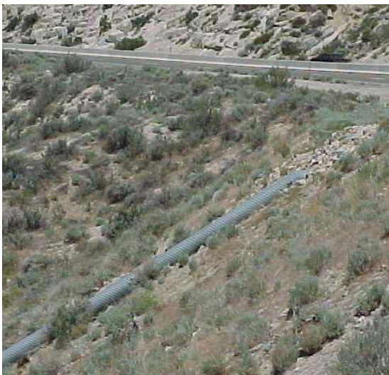
Figure 2.25 Culvert slope drain.
