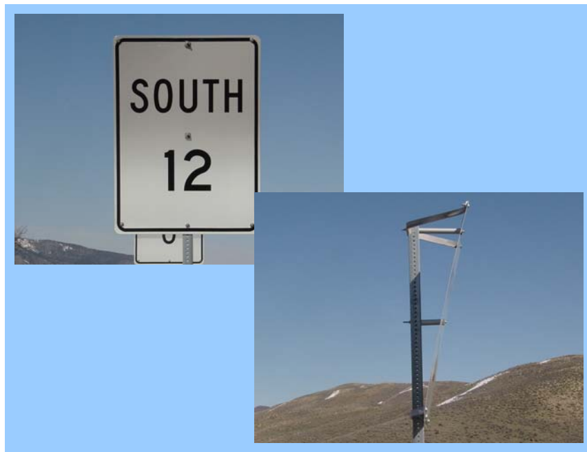
Figure 2-3. Illustration of Vertically Tilted Sign Installation
