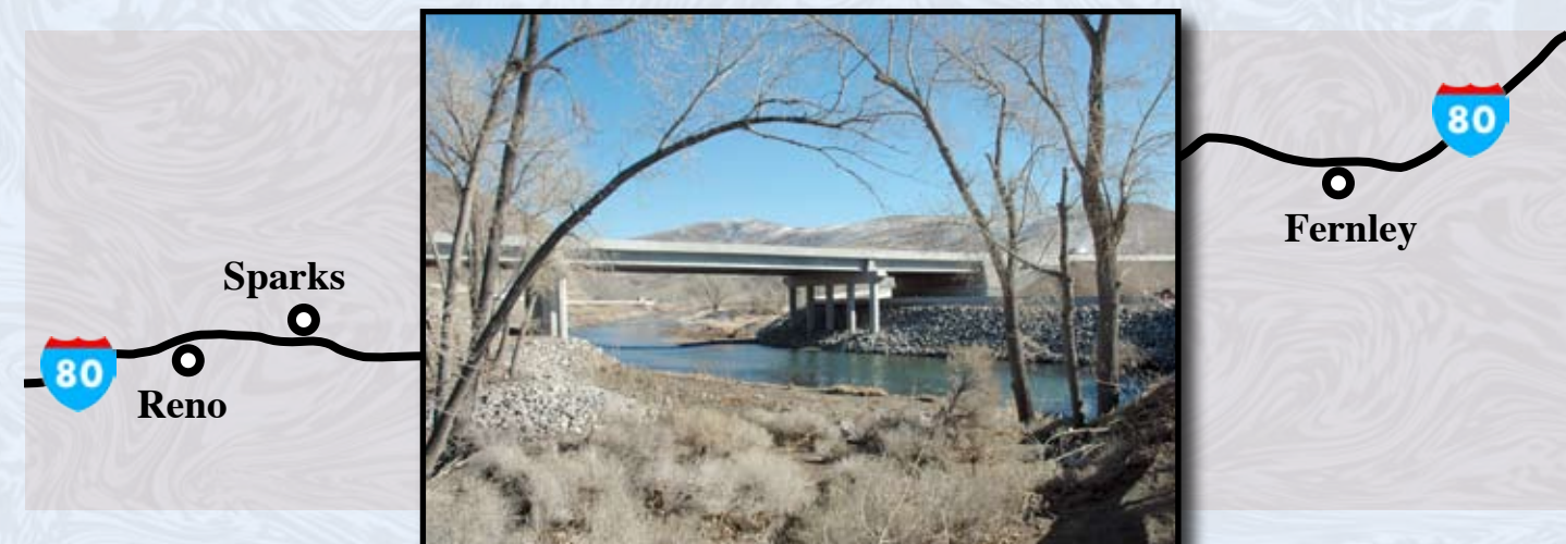
Interstate 80 traffic can be seen running behind the Truckee River bridge portion of the new USA Parkway interchange.
