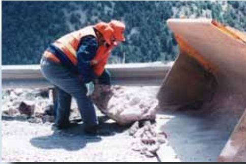
Removing Boulder
