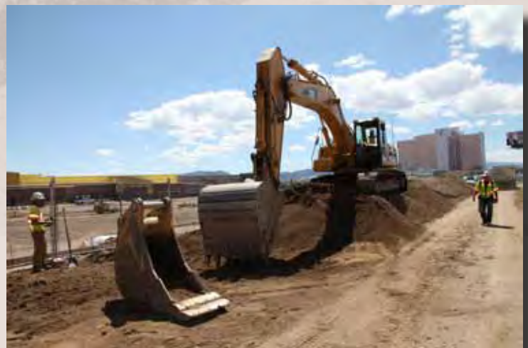
Construction gets underway on the northbound U.S. 395 project.
