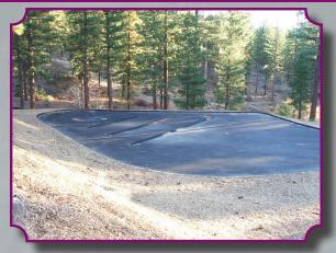
Heavier sediment is deposited as wastewater slowly drains in the Incline Village decant basin on its way to a treatment plant.
