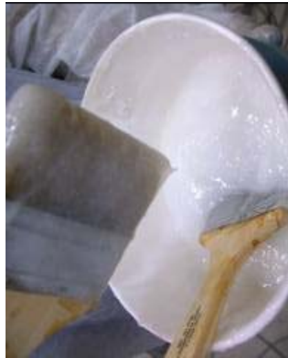
(d) Thickening epoxy with cab-o-sil prior to vertical application to blocks
