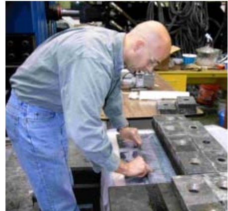
(b) Squeezing Excess Epoxy from Fabric
