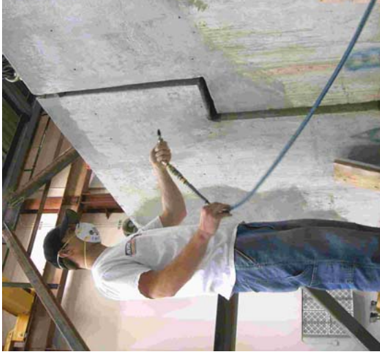
(b) Air-blasting prior to restrainer attachment
