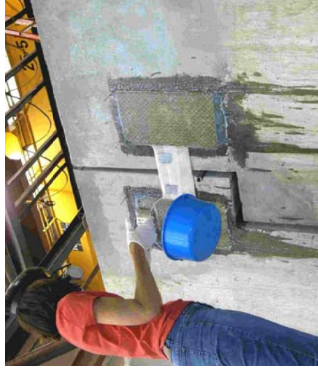
(e) Second coating of epoxy
