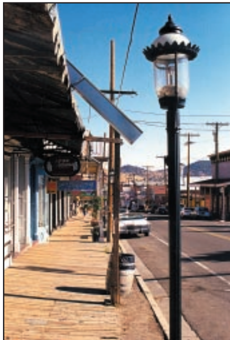
Virginia City's street lighting project will be extended with enhancement funding.
