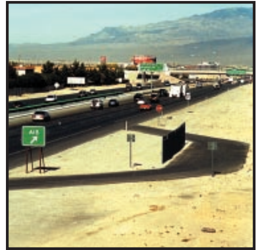
Accident investigation sites free up shoulders on U.S. 95.
