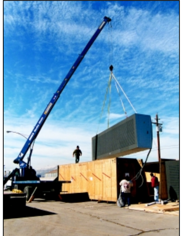
OUT OF THE BOX—A crane lifts the Dambach dynamic message system out of its crate at the NDOT yard in Reno and loads it onto a flatbed truck. Next stop is a sign bridge and installation.
