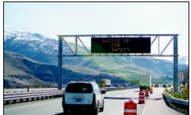
UP AND WORKING—Starting with a test message, the changeable sign westbound on I-80 near Mogul will provide valuable information for travelers, alerting them to road and weather conditions ahead.
