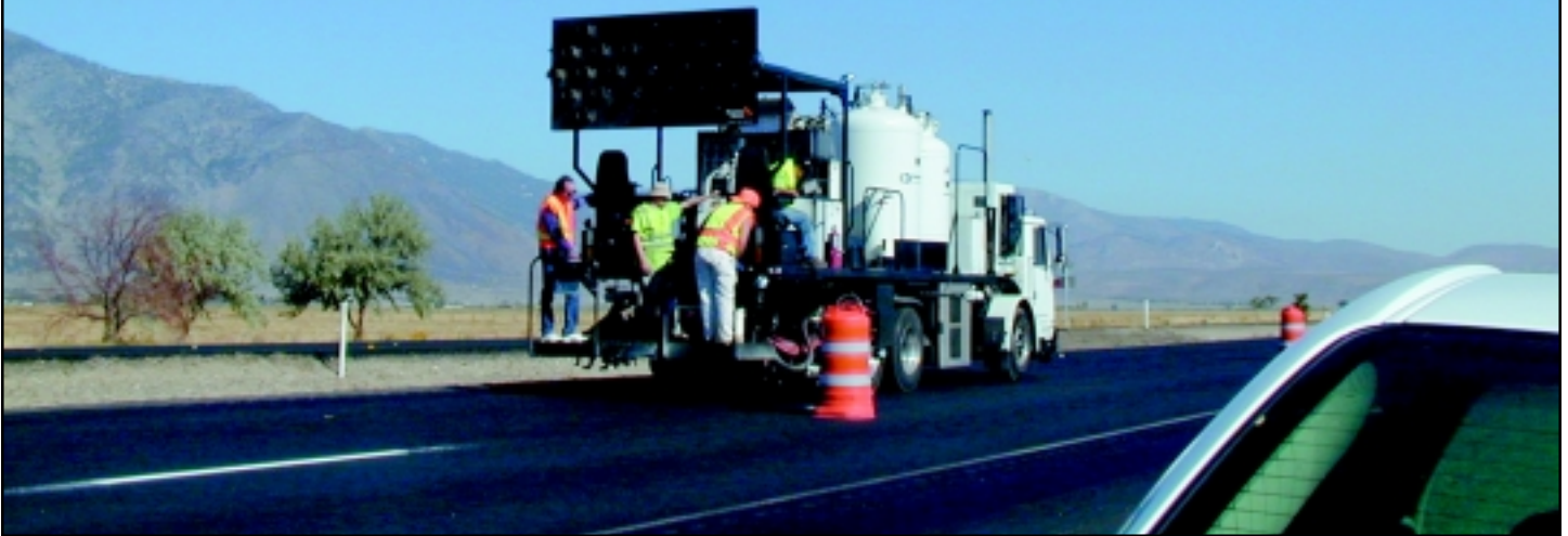
APPLICATION—A type of polyurea marking material is applied to the roadway south of Carson City. NDOT Research and Development will monitor how the pavement marking performs under actual traffic conditions.
