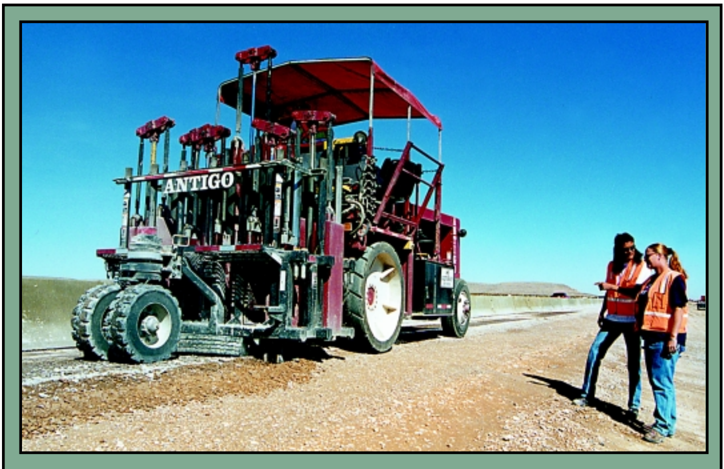
Top left: Concrete cracking begins with a saw making a clean cut to protect remaining concrete.
