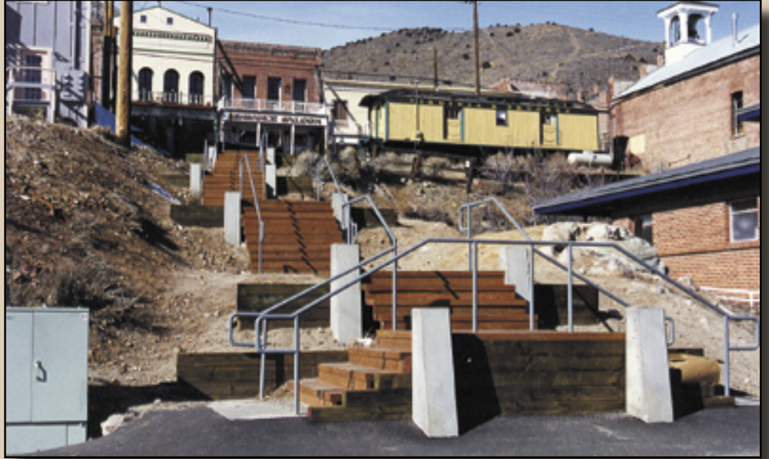
COMSTOCK CLIMBERS—Helping to preserve the Old West flavor of Virginia City, an enhancement project assisted with planning for restoration of a boardwalk, gas style electric lights and kiosks.
