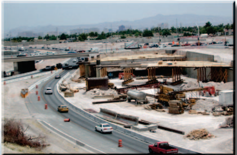
RAINBOW CURVE—NDOT is widening US-95 in northwest Las Vegas. The $42 million project will include the freeway from four to six lanes from Rainbow Boulevard to Craig Road.
