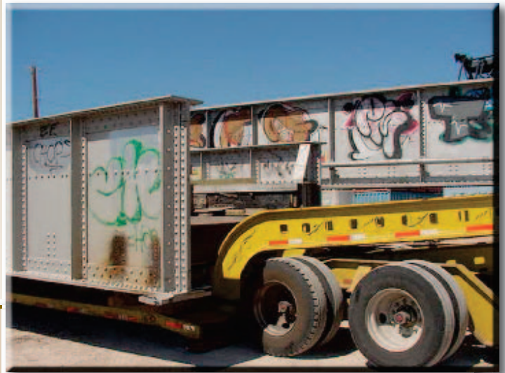
LOWBOY--Sections of the former Union Pacific Railroad bridge have been loaded on trailers to be moved north.
