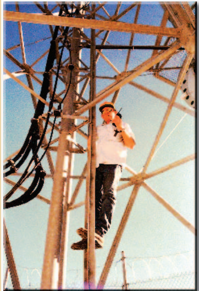
ANTENNA MAN—Jim Kraus takes a call prior to working on equipment located on Mt. Brock above Tonopah. The cooperative statewide radio network provides excellent service for public agencies and others.
