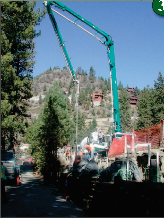
DURING—A cement snorkel truck delivers material where needed.
