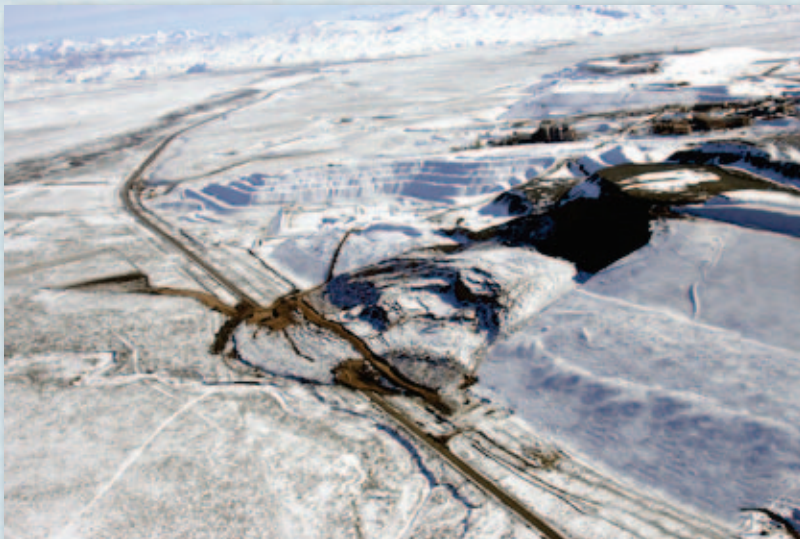
BIG SLIDE—This aerial photo shows hundreds of thousands of tons of rock and earth on top of SR-766 near Elko in early February. The slide has since been excavated and the road was scheduled to be re-opened.--Photo courtesy Ross Andreson, Elko Daily Free Press
