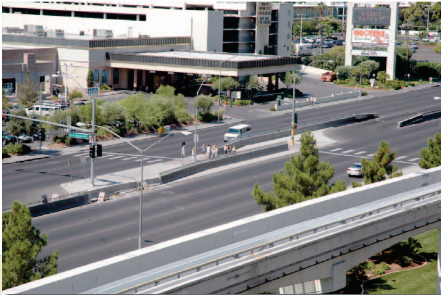
INNOVATIVE--A short pedestrian crossing light and the need to keep walkers from crossing Tropicana Avenue against the signal led to the innovative approach shown above. Those crossing the busy Las Vegas street cross halfway with one light and cross the second half at a second signal. The setup creates better traffic flow and protects pedestrians.
