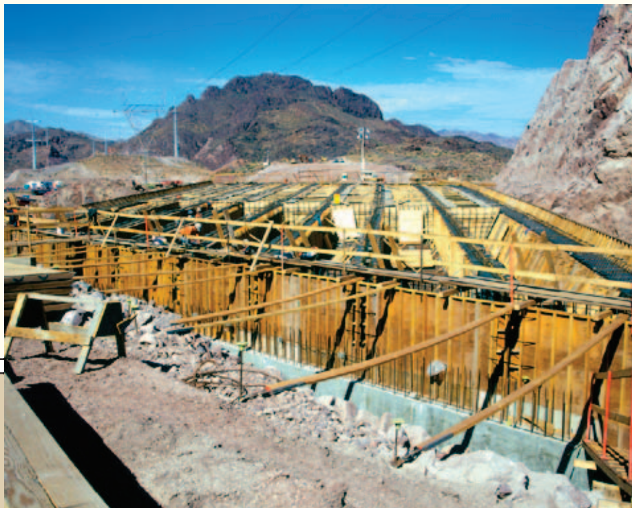
IN PROGRESS—View of Edward Kraemer & Sons constructing formwork for the girder sections at the Old US-93 overpass. Photo courtesy of FHWA.
