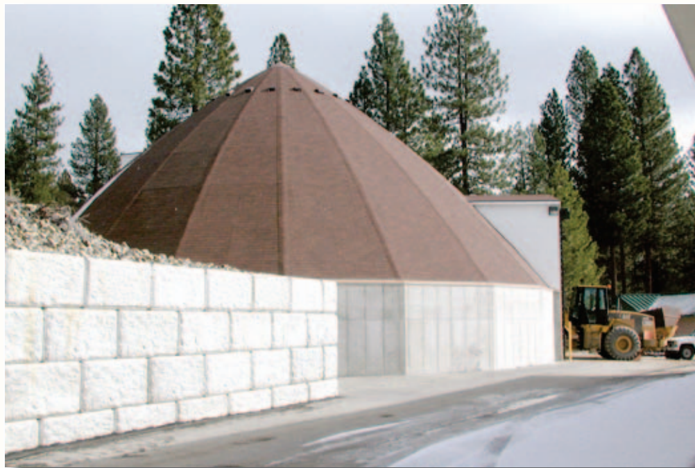
To preserve NDOT's sand and salt piles and to keep them from leaching into the environment, more domed structures are being used around the state.
