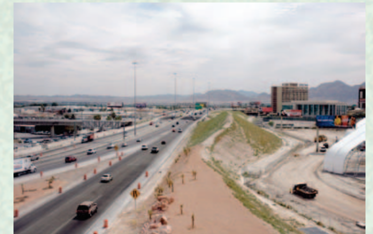
I-515—One of several corridor studies is I-515 from the Spaghetti Bowl in Las Vegas to Foothill-Eastern and Southeast.
