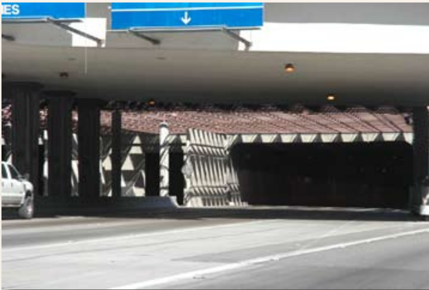
AIRPORT CONNECTOR--The first section of the Southern Beltway (I-215), from I-15 to McCarran Airport, along with a connecting tunnel beneath the east-west runways, was opened to traffic in 1994.
