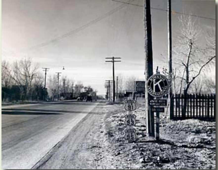
FABULOUS LAS VEGAS—Instead of a blaze of neon, a concrete road and a gentle change from rural to urban mark the entrance to Las Vegas in the 1940s. Note the sign marking all the interstates.
