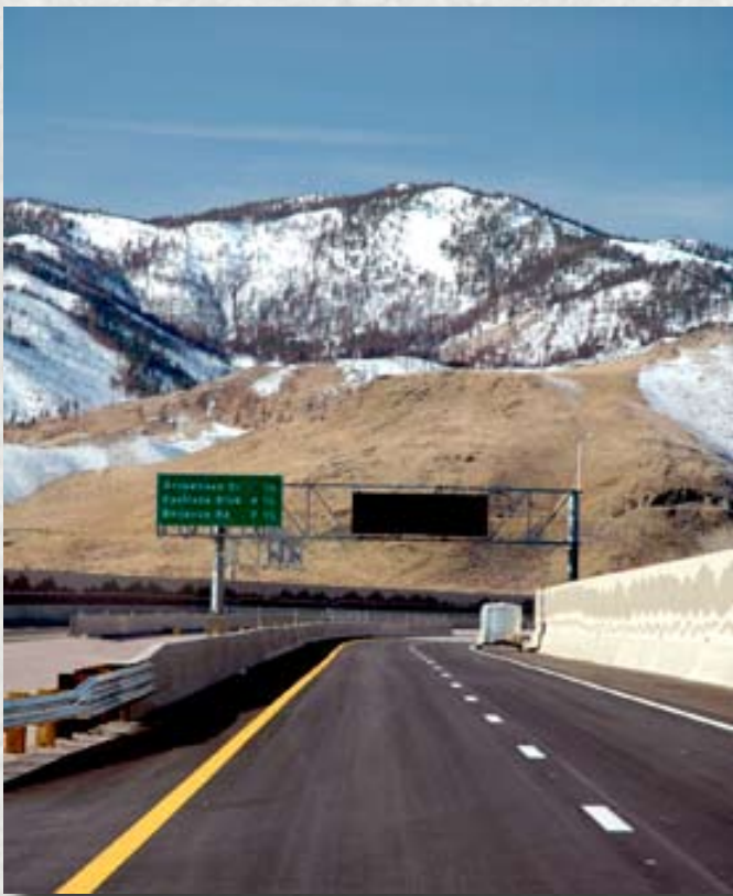
READY TO GO—Just before opening to vehicles in February, the Carson City Freeway has a Dynamic Message System sign in place, freeway signs and bright new striping. The Carson City Freeway is one of six Nevada “super projects” designated in the 1990s.
