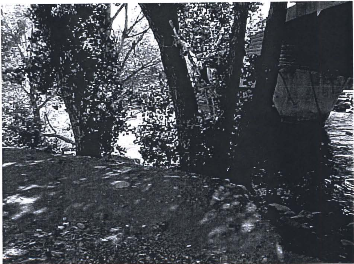
Kuenzli bridge from west bank looking east.
