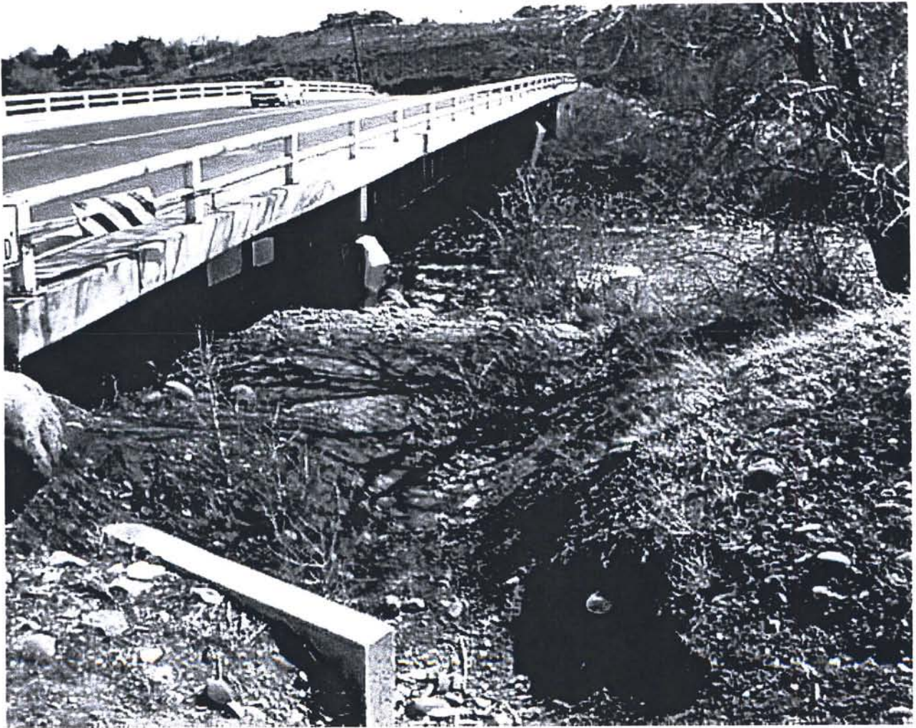
Mayberry Bridge – NW Corner (looking south)
