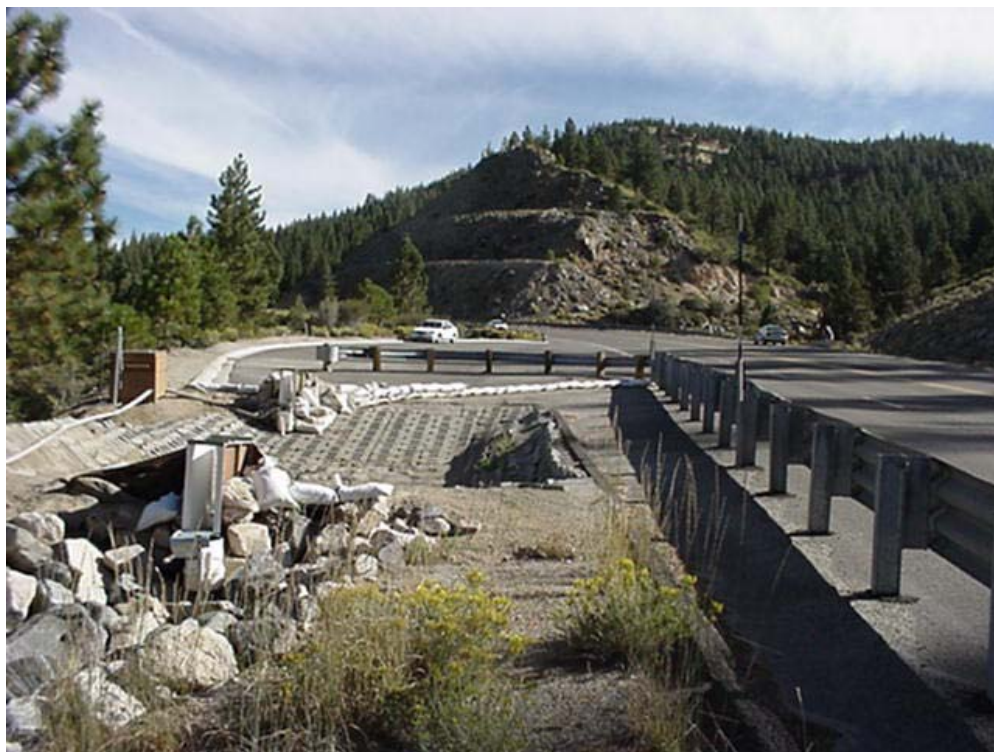
Figure 6.1. NDOT 3, U.S. Highway 50 sediment basin.
