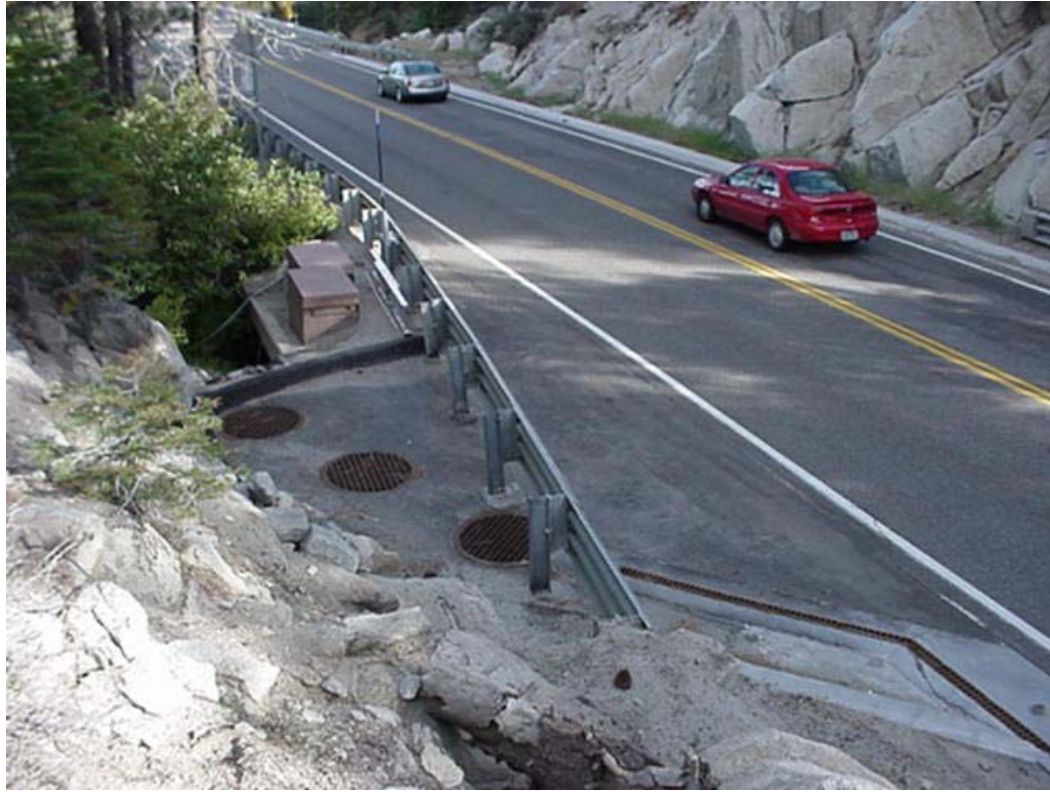
Figure 4.2. Triple-barrel sediment trap at Secret Harbor Creek.
