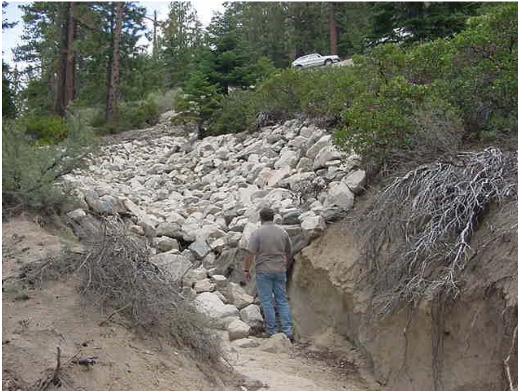
Figure 9.1. Riprap channel terminus on steep hillside below SR 28.
