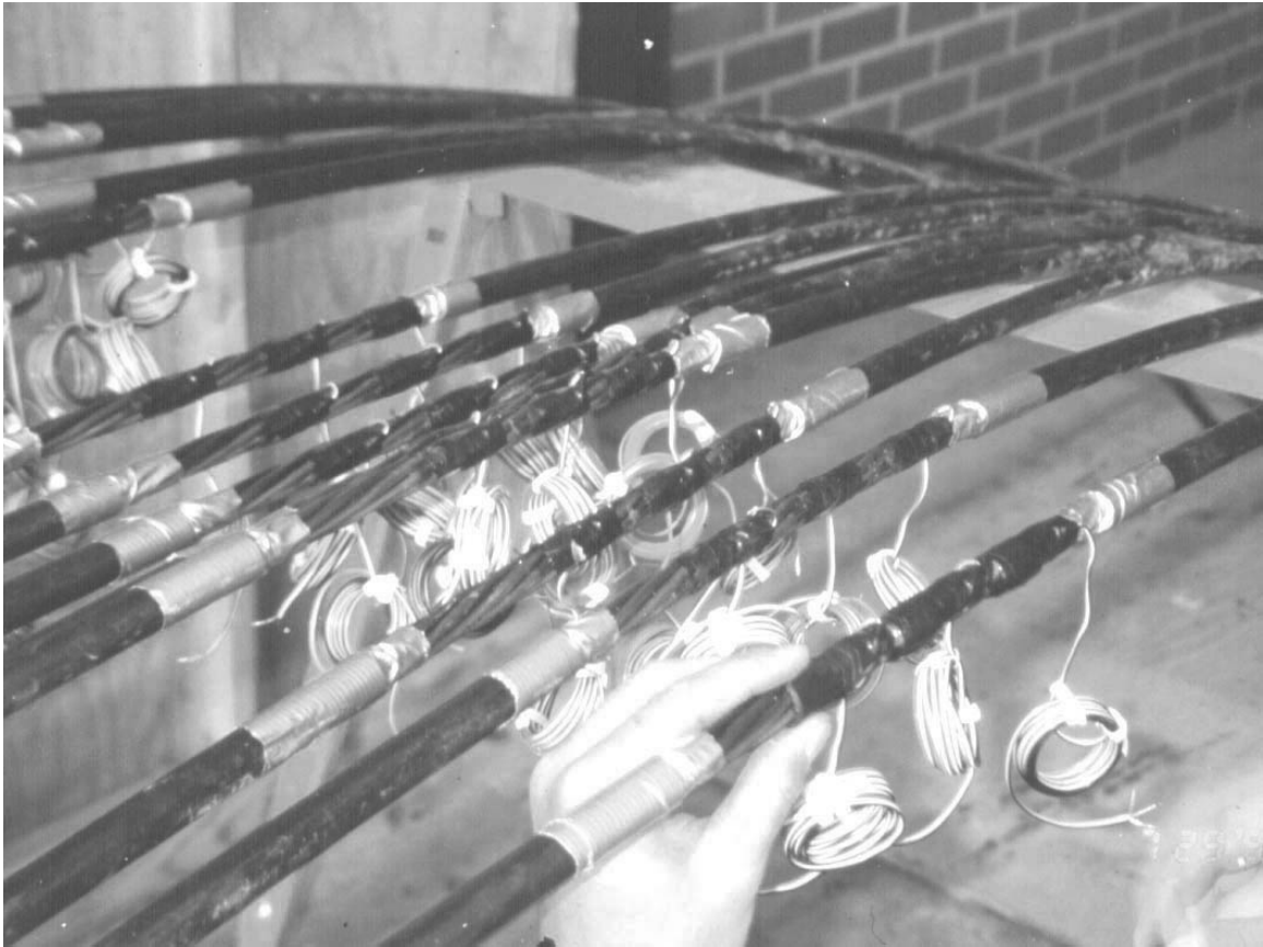
Figure 3.2 – Strain Gages on Box Girder Tendons
