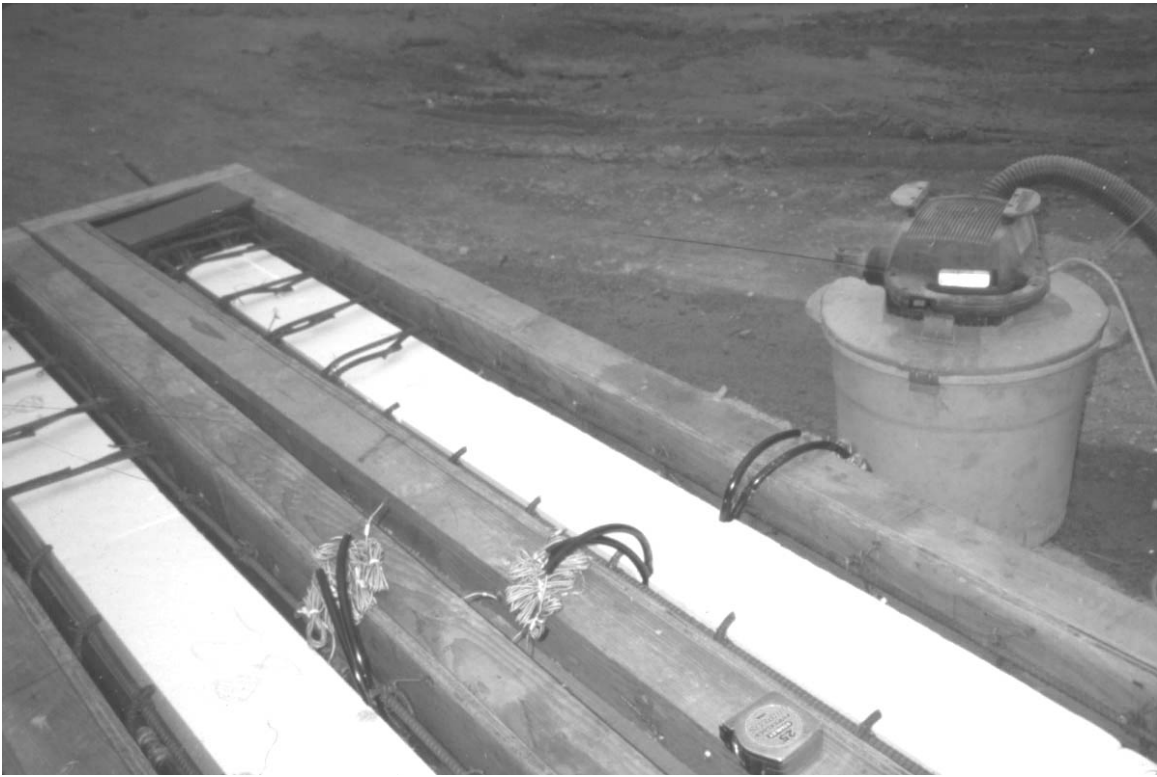
Figure 2.5 – Box Girders Under Construction
