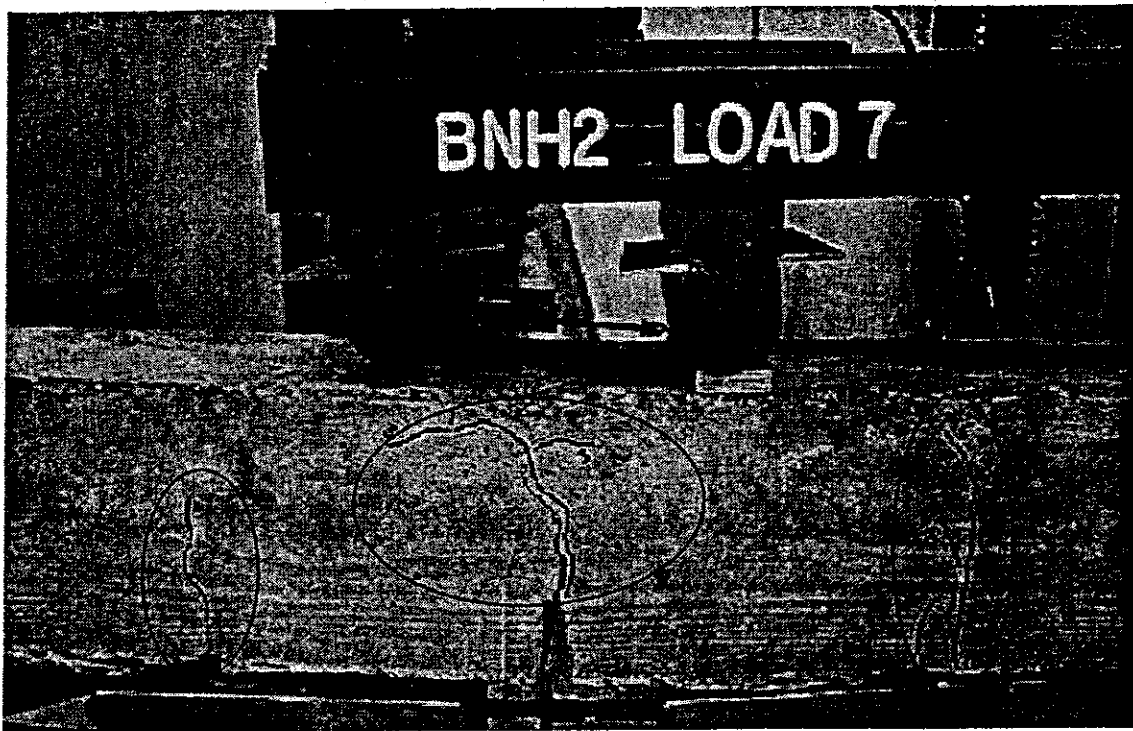
Figure 3-52: BNH2, Failure after final Cycle 7
