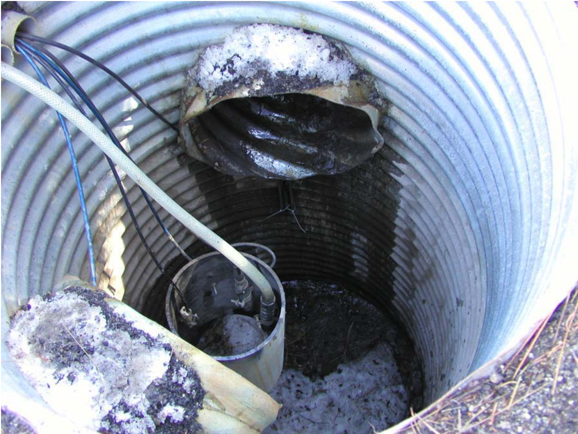
Figure 3.2. Sample collection tube, temperature, EC and turbidity sensors within sediment trap at NDOT 2.
