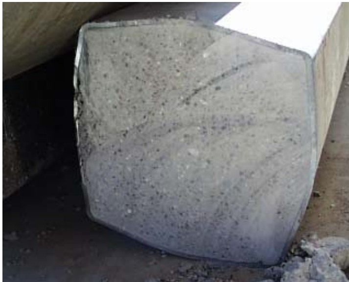
Figure 3-6: Cross-section of Steel Tube with the Grout Mix Design containing 8.5-sack of Cement, Section III
