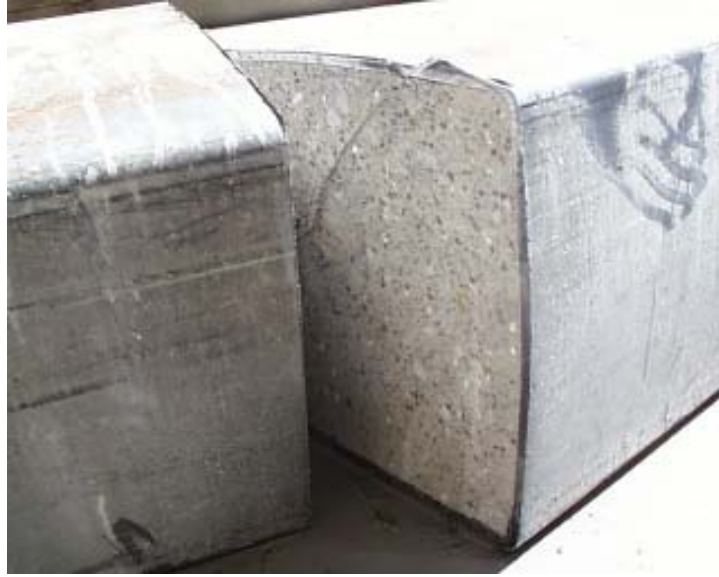
Figure 3-7: Cross-section of Steel Tube with the Grout Mix Design containing 8.5-sack of Cement, Section IV
