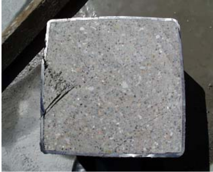
Figure 3-5: Cross-section of Steel Tube with the Grout Mix Design containing 8-sack of Cement, Section V
