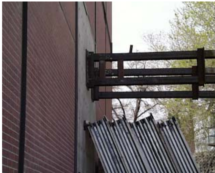
Figure 2-15: Actual Steel Frame Mounted to Wall
