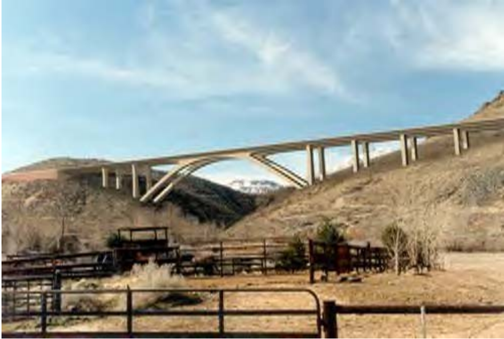
Galena Creek Arch Bridge over Galena Creek.
