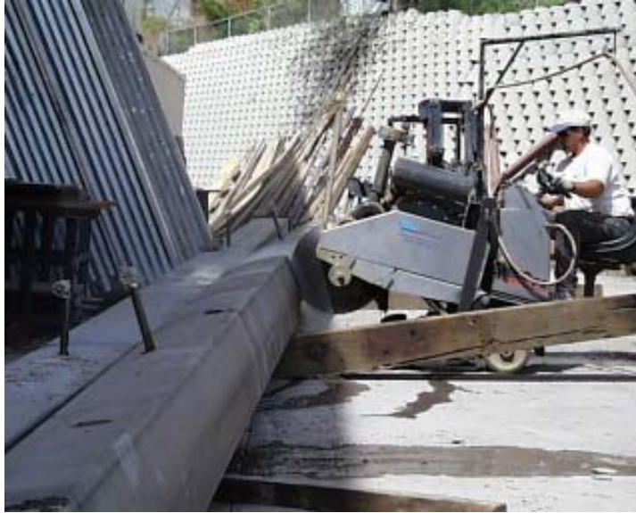
Figure 3-9: The Structural Steel Tubes Starting to Get Cut
