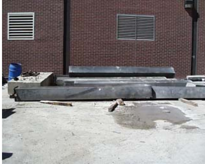
Figure 3-11: The Structural Steel Tubes Cut in 15-foot Segments
