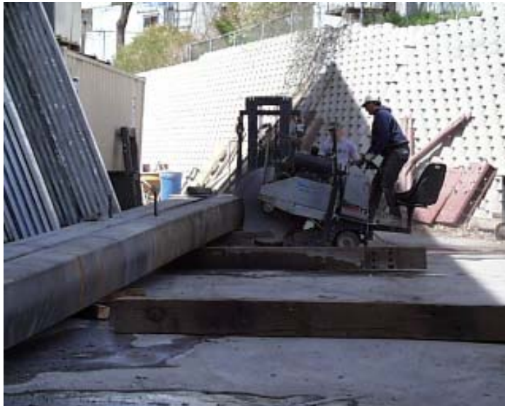
Figure 3-10: The Structural Steel Tubes Being Cut with the Larger Blade
