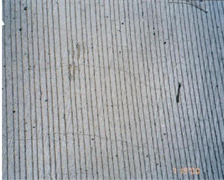
**Figure 3-5. Longitudinal cracks under wheel paths on the North bound lanes of the I-1951 Zolezzi structures. Mild shrinkage cracks were observed over the entire deck.**
