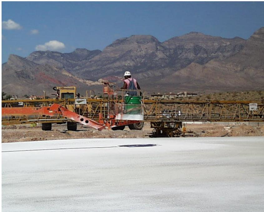
**Figure 3-7. (a) Sahara deck crack photographed eight hours after deck pour; (b) curing compound being applied eight hours after deck pour.**
