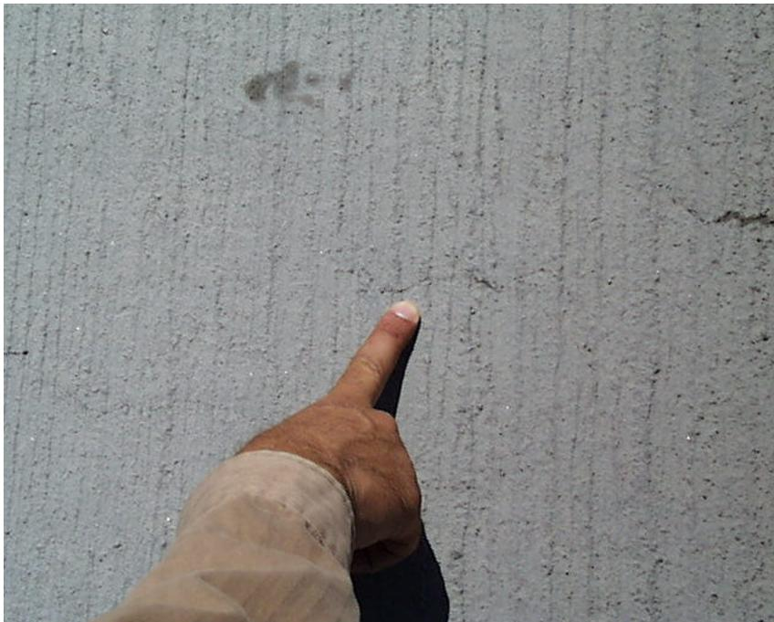
**Figure 3-10. (a) Overall view of the Desert Inn Bridge; (b) the only visible surface crack on the whole deck.**
