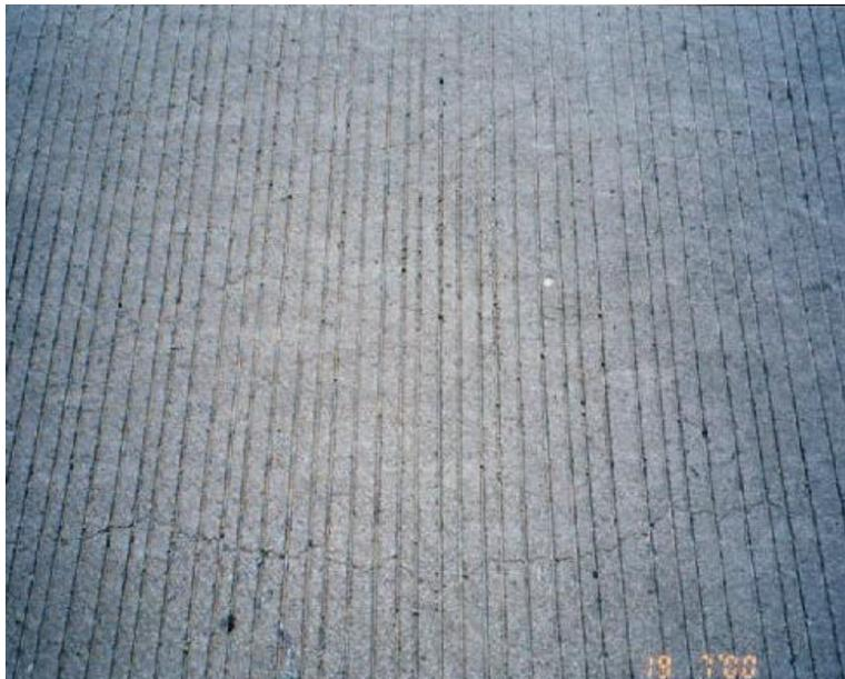
**Figure 3-6. Shrinkage cracks of the I-1305R Clear Acre slip ramp. Entire deck was in fair to good condition. Deck and approach slab are monolithic, and approach slab had more**
