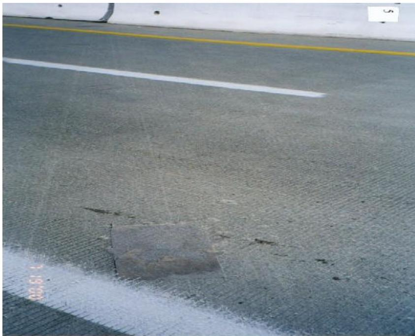
**Figure 3-4. (a) Transverse and longitudinal shrinkage cracking following the pier caps of the Mt. Rose and I-580 Bridge; (b) transverse cracks over the pier caps.**
