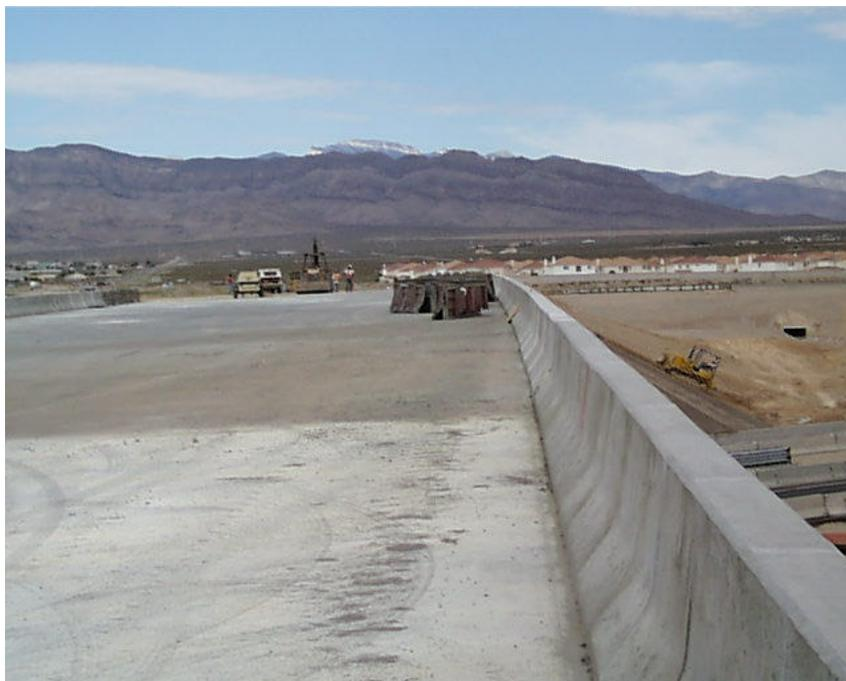
**Figure 3-9. (a) Extensive cracks in the mid-section of the deck; (b) finished deck two months after deck pour. A difference in surface color indicates sections separation during the three-section deck pour process from July 5 to July 6, 2000.**
