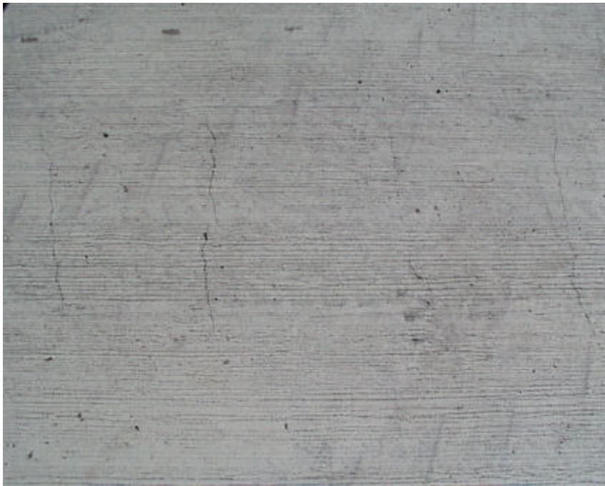
**Figure 3-3. (a) and (b) Longitudinal and diagonal cracks on the Steamboat Creek bridge deck.**
