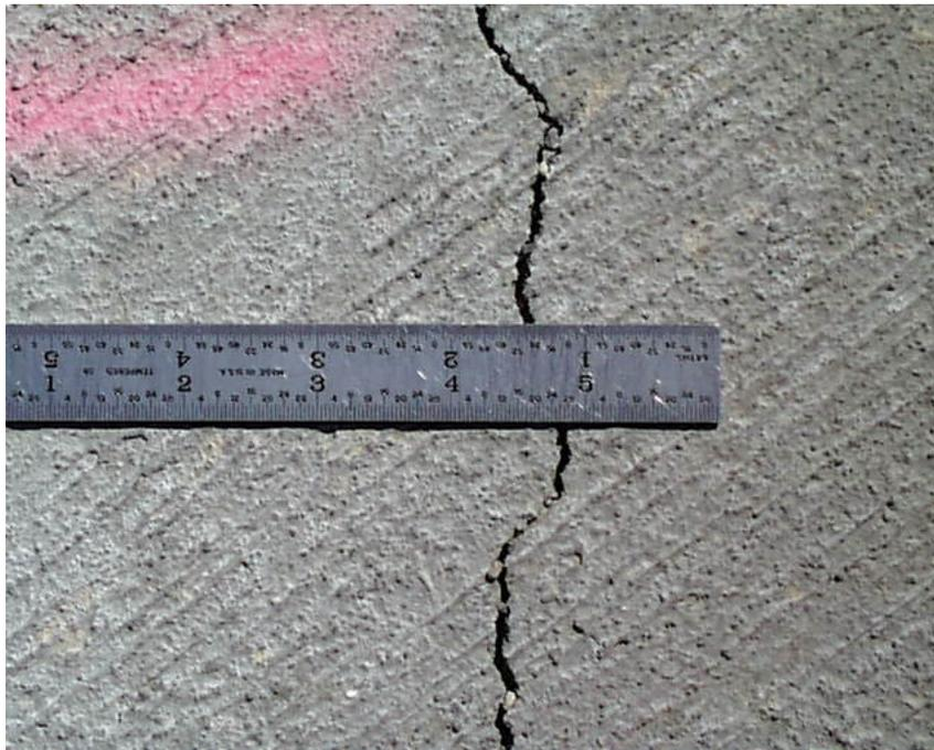
**Figure 3-8. (a) and (b) show combination of longitudinal and transverse cracking on the U.S. 95 Highway bridge deck project.**
