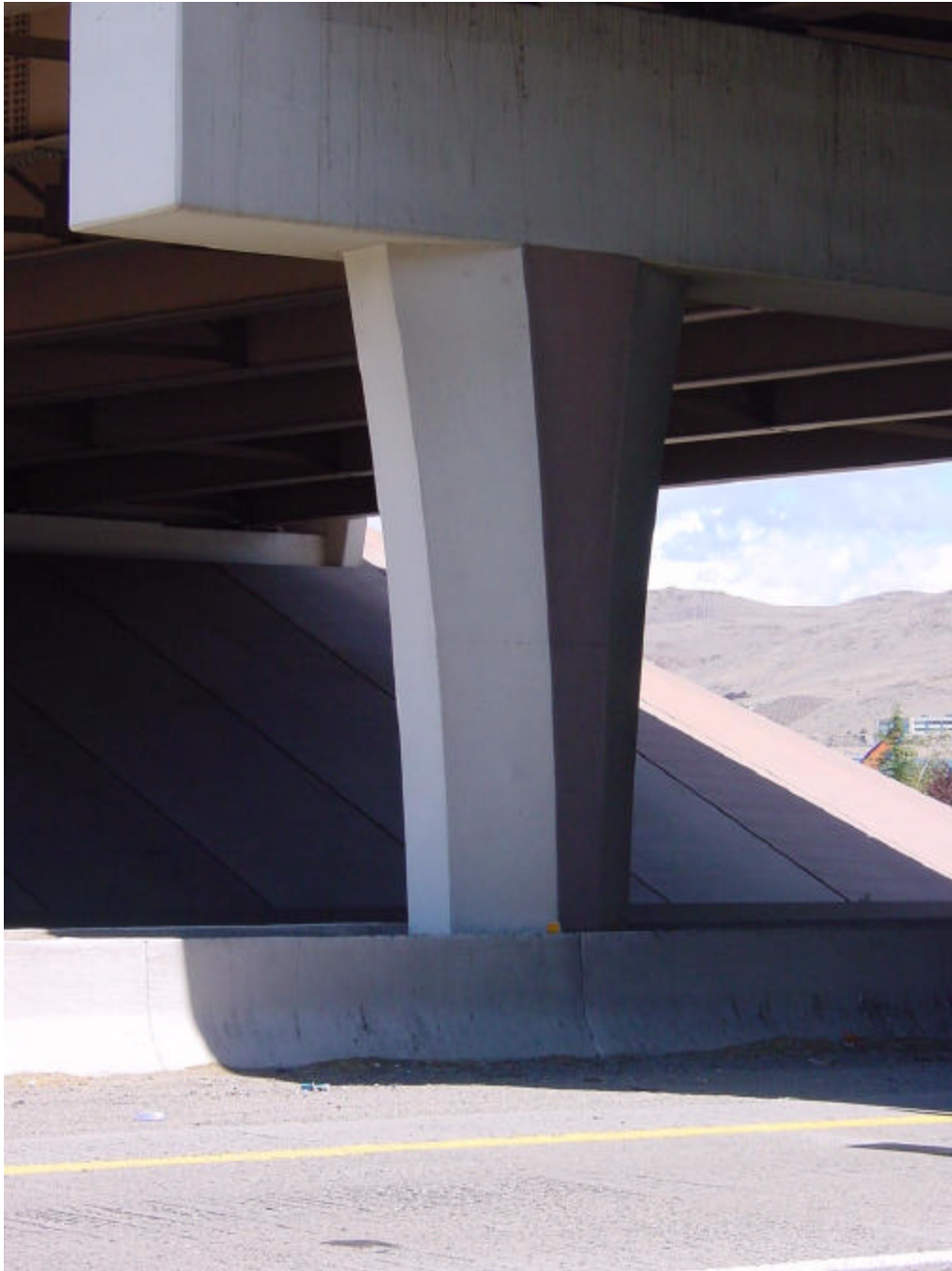
Figure 2 - 1 A View of the Edge Column in Bridge I-1556
