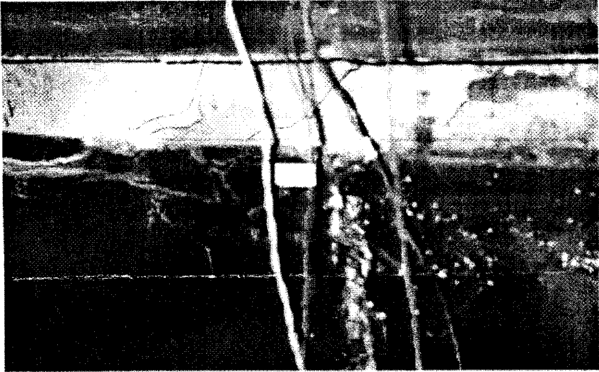
Fig. 3-37 Specimen FR, Run 8, Cracking
