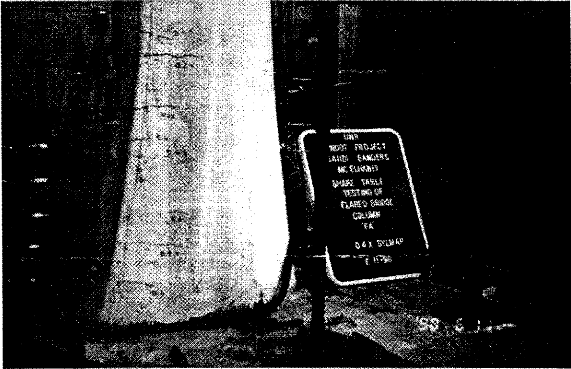
Fig. 3-11 Specimen FA, Run 2, Cracking
