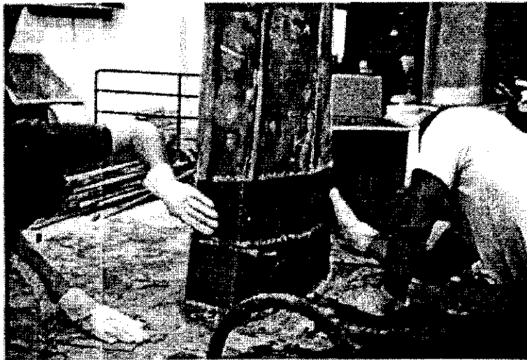
Figure 2 - 12 Composite Fabric Installation
