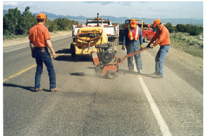
Routing for crack sealant installation.
