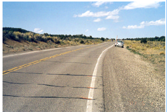
Crack sealant test site on S.R. 278 near Eureka, Nevada.
