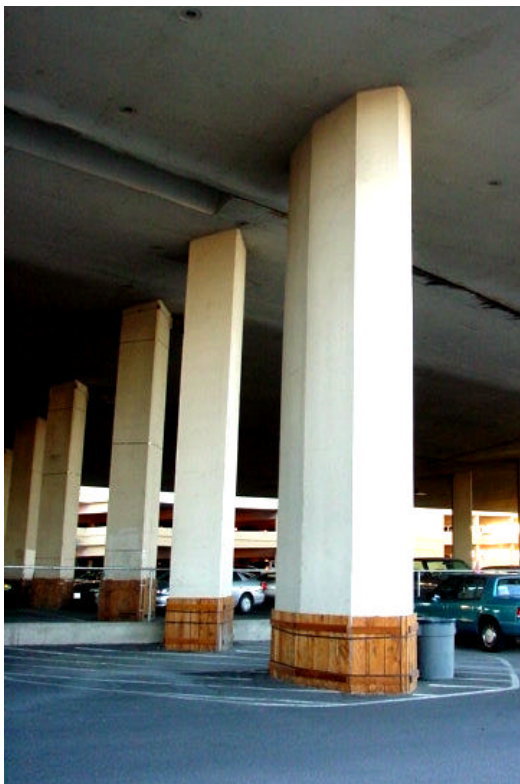
Fig. 1 Elevation view of octagonal and diamond shape columns.
