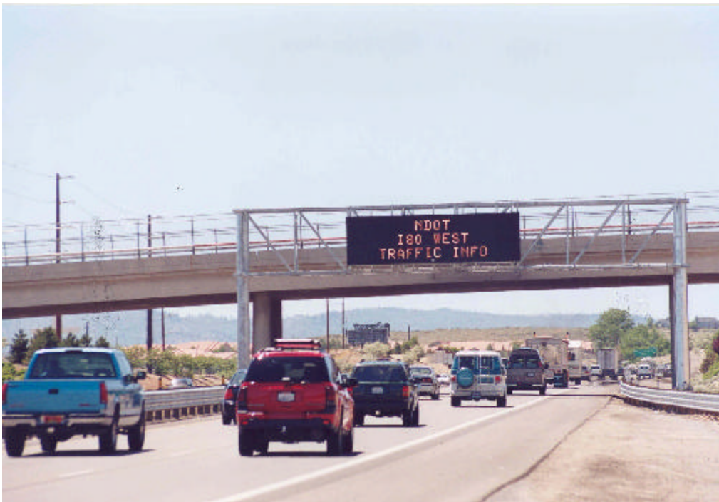
Photo 3. Dynamic Message Sign helps to inform motorists of road conditions and traction device requirements ahead on westbound I-80 over Donner Pass.
