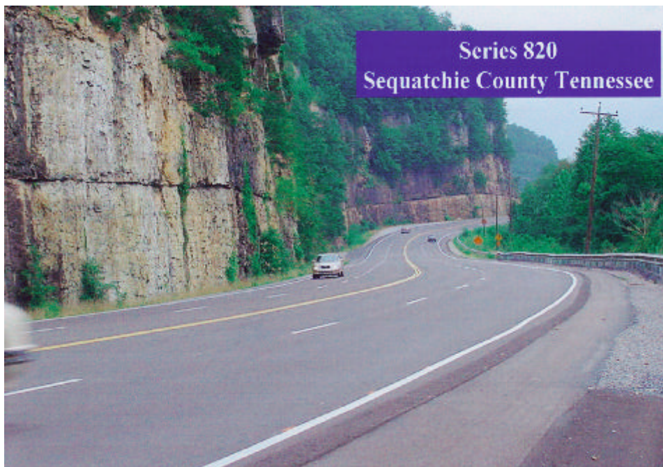
Photo 2. Wet reflective tape series 820 installed in Sequatchie County, Tennessee.
