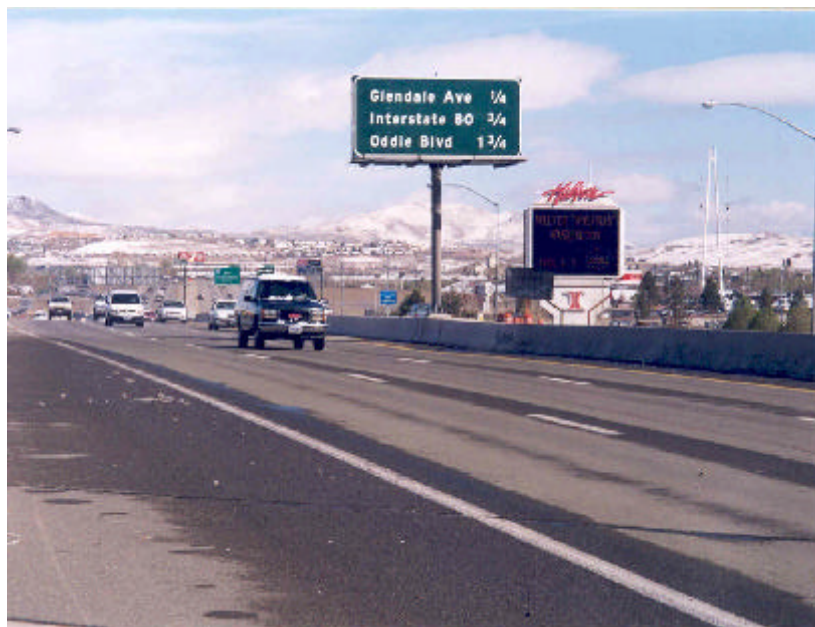
Photo 1. Thin epoxy overlay systems being tested on US 395 in Reno.
