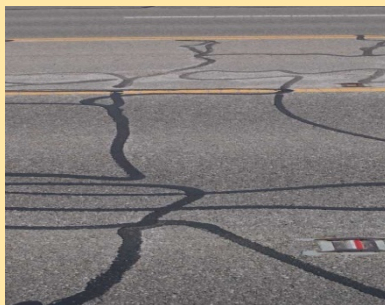
Crack Sealing
