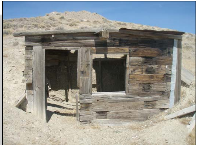
Railroad tie construction, Double O Mine site. Photo by Sena Loyd.
