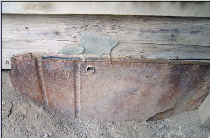
Automobile door panel reprioritized to repair dugout wall in one of the features, Double O Mine site. Photo by Sean McMurry.
