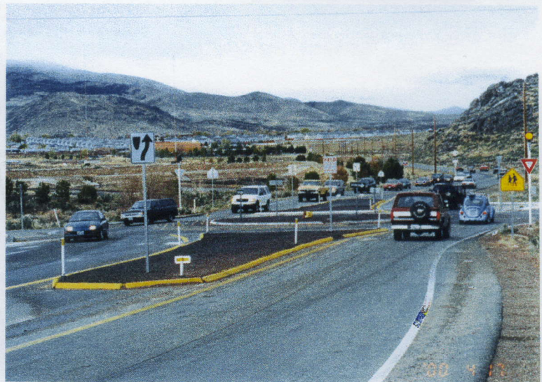
Roundabout on Edmonds Dr. and Fifth St.
