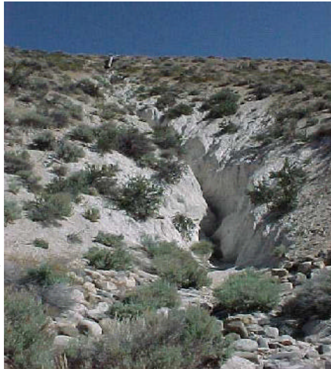
Photo 1: Severe erosion along U.S. 50 resulting from a culvert with free discharge.
