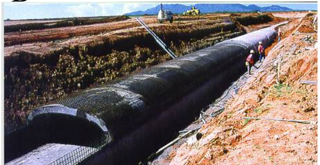
Photo 3. Constructing Con-Arch culvert system
