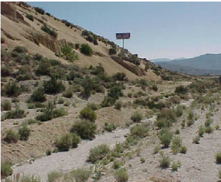
Photo 2: Erosion along U.S. 50 is exacerbated by steep slopes and shallow soil profiles.
