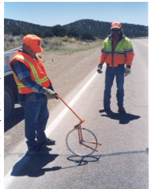
Figure 1. Measuring crack length.
