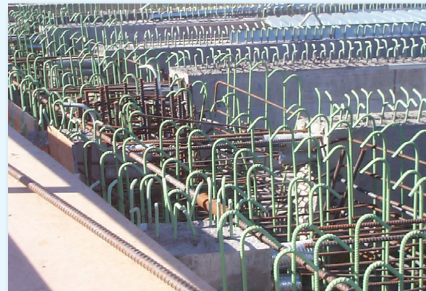
There, that should be enough rebar
