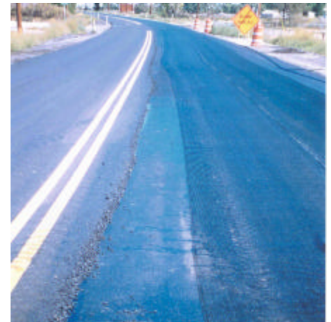
Photo 7. Completed installation of GeoGrid fabric prior to asphalt overlay.
