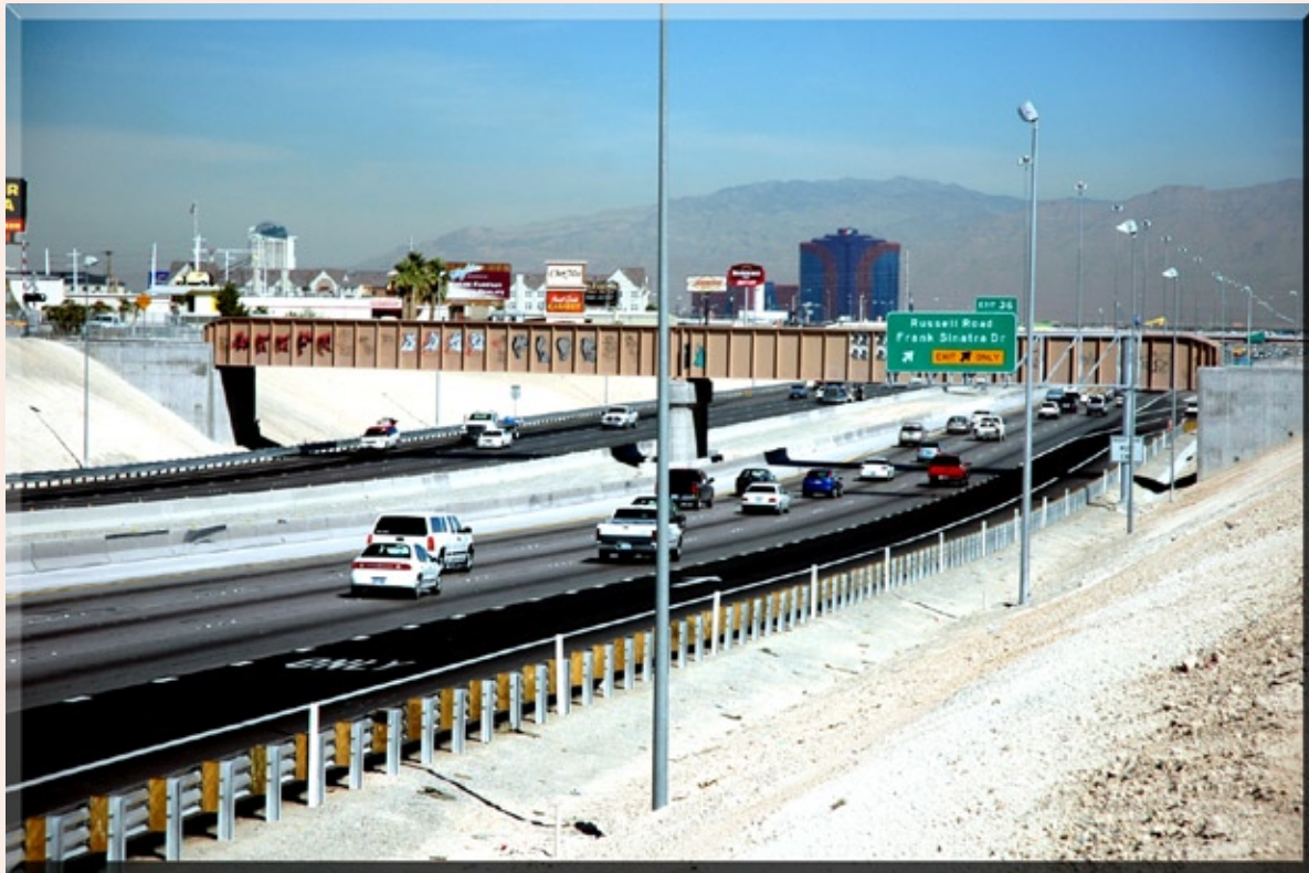
VANDALIZED--As soon as this railroad bridge was erected over I-15 in Las Vegas in early 2004, graffiti vandals went to work, defacing the structure. NDOT has a full-time crew of 10 plus two supervisors who paint out graffiti, pick up trash and assist in landscaping projects.
