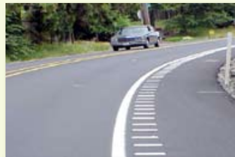
Raised Rumble Strips
