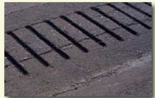
Rolled Rumble Strips
