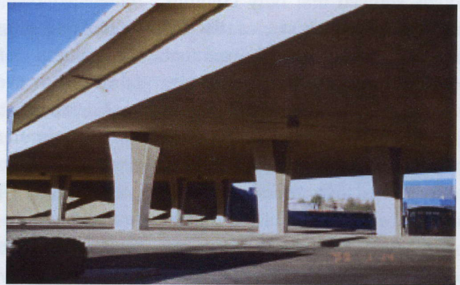
Typical columns with structural flares in Nevada bridges
