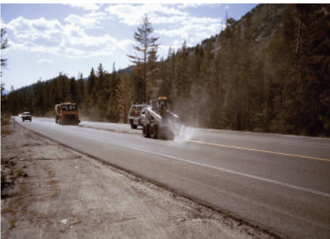
Photo 1. Equipment Grinds out a Swath to Inlay Products on SR 431.
