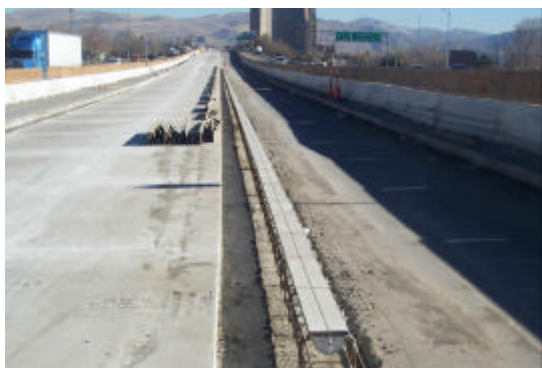
Photo 3. The Trench Drains Installed on I-80 Project in Sparks.
