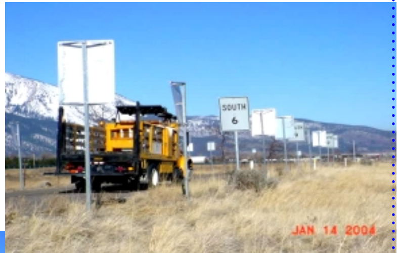
Signs installed facing different directions
