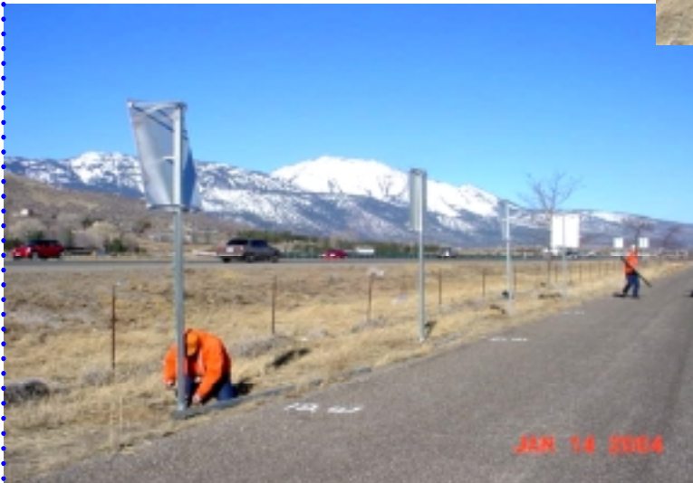
Signs being installed at Washoe Valley
