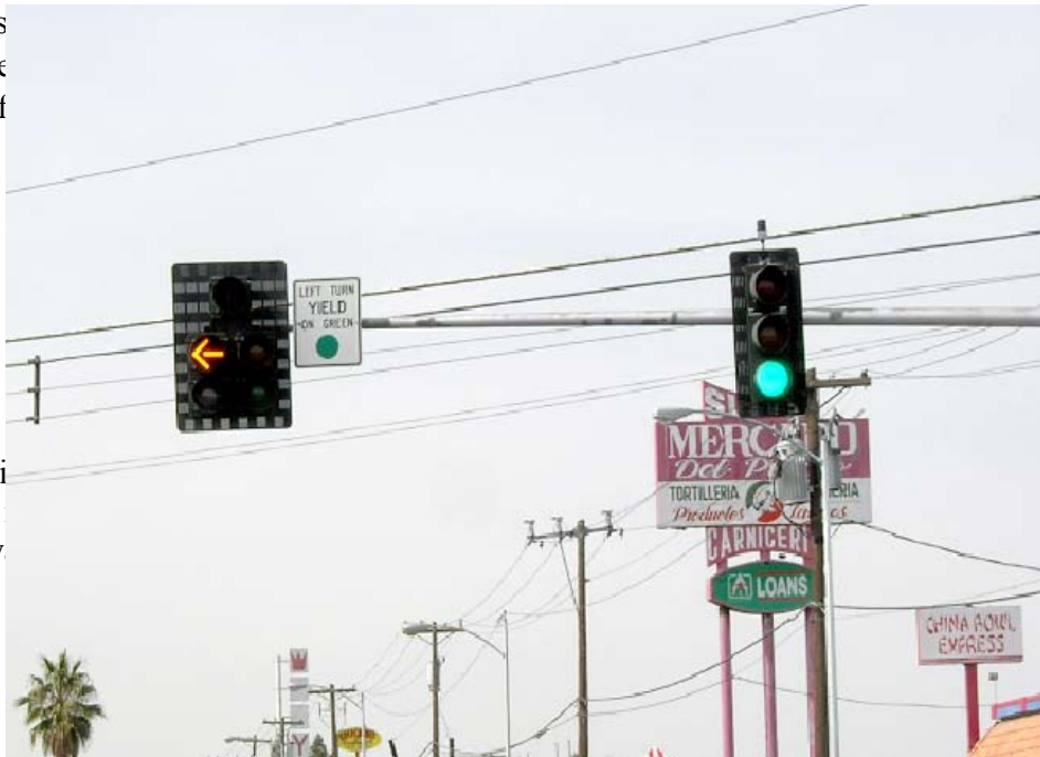
Figure 3: Illustrates the special time-of-day protected/permitted left-turn
