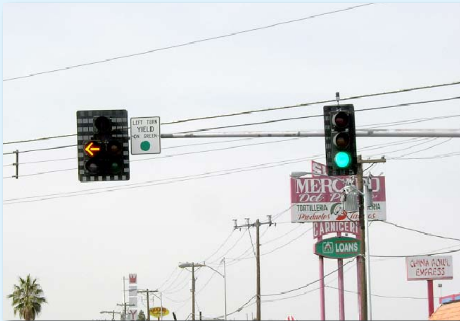
Figure 3: Illustrates the special time-of-day protected/permitted left-turn operation in Las Vegas. The left-turn signal head with the protected/permitted design operates protected-only during the peak periods by turning off the lights for the permissive green ball and yellow ball that allow the permitted left turn movements during the off-peak periods. The yellow arrow display, during a peak period, indicates that the protected left turn movement is about to terminate.
