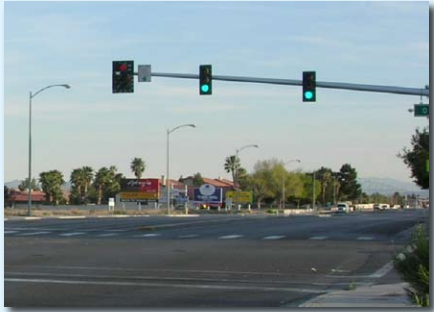
Figure 2: Shows the typical protected left turn display with a red arrow. With a green arrow, a driver has the right-of-way to make a left turn.
