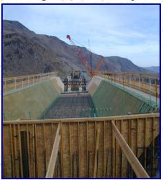
A taller, 42-inch barrier rail will be employed along the entire length of the I-580 Freeway Extension corridor as opposed to the standard 32-inch barrier rail typically used. This
