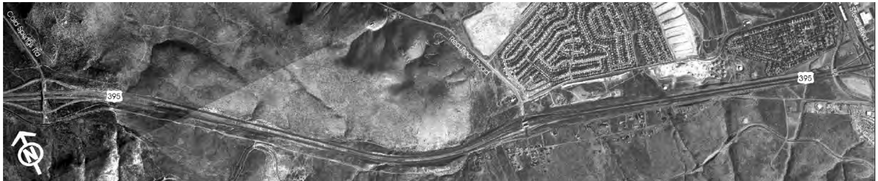
Figure 2-13: US-395/I-580 from Cold Springs Road to Stead Boulevard
