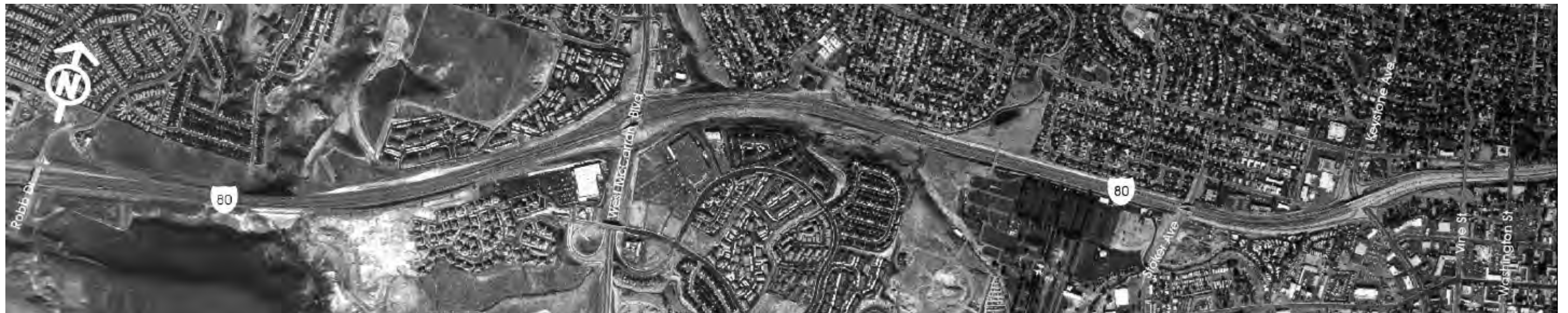
Figure 2-10: I-80 from Robb Drive to Washington Street
